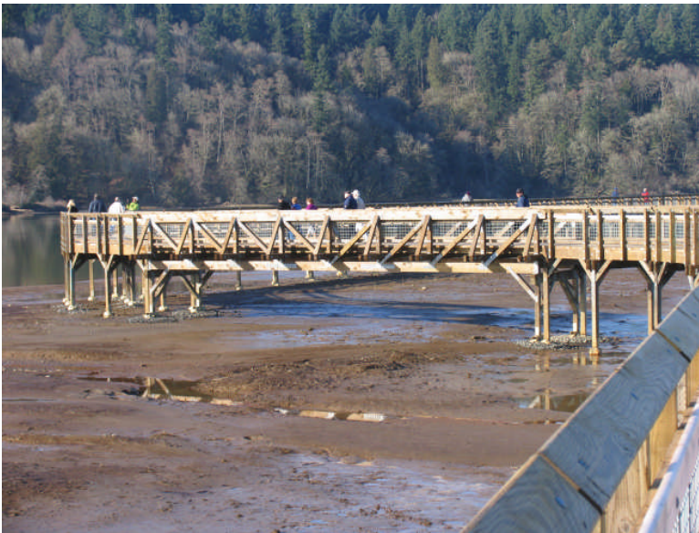
Figure 6. 15.24m (50'-0") Pony Truss Bridge
