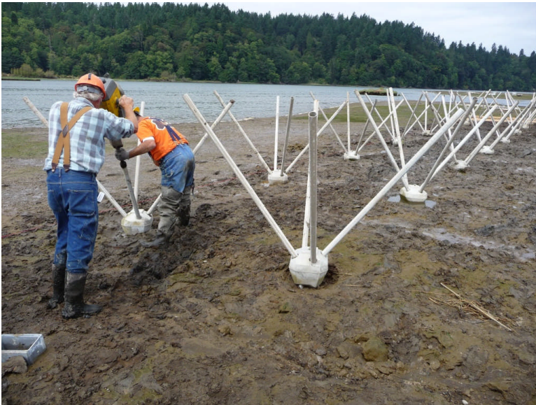
figure 2. Installation of Diamond Piers.
