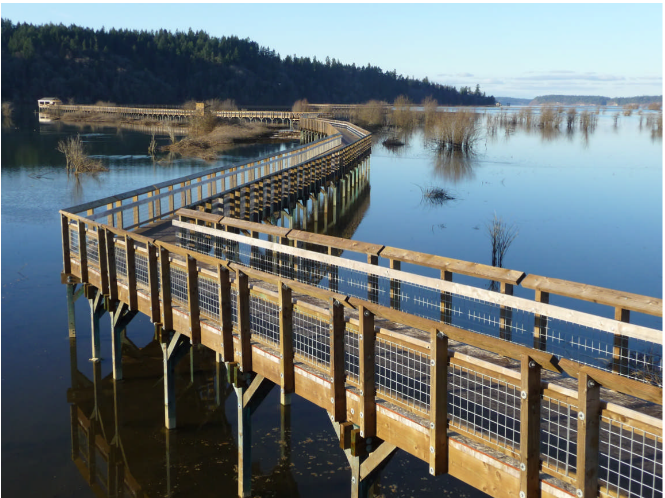
Figure 7. Boardwalk at high tide with bird viewing blind and viewing platform
