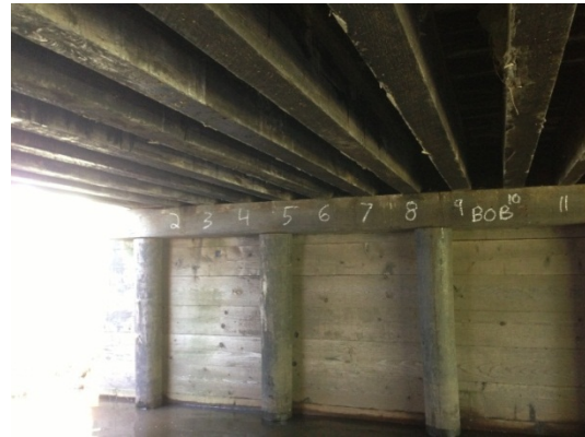
Fig. 5 Timber girder bridge underside view from Cluster 2 in Blackhawk County
