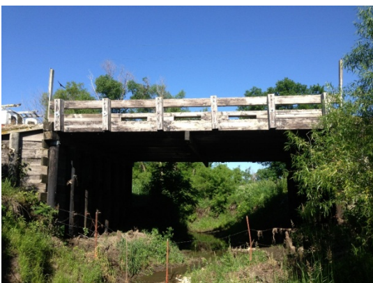
Fig. 6 Timber deck bridge elevation view from Cluster 3 in Clarke County
