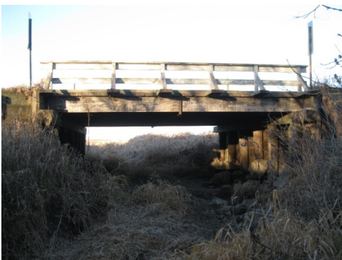
Fig. 2 Timber girder bridge elevation view from Cluster 1 in Bremer County
