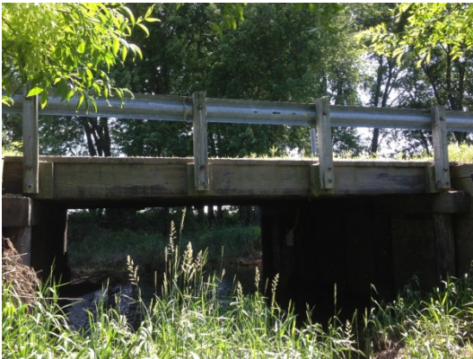
Fig. 4 Timber girder bridge elevation view from Cluster 2 in Blackhawk County
