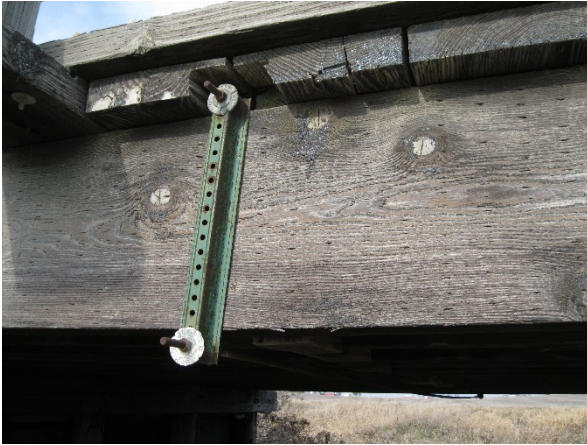
a. Exterior tension rod connection
