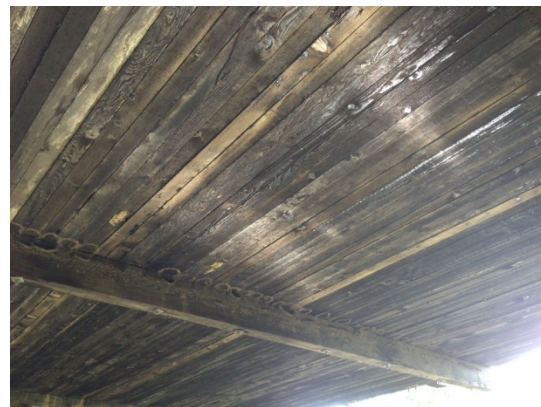
Fig. 7 Timber deck bridge underside view from Cluster 3 in Clarke County
