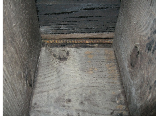
b. Tension rod between girder and deck
