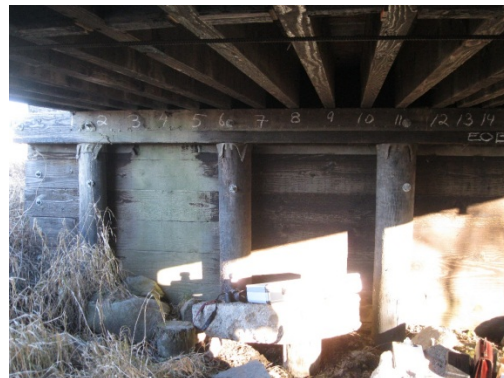
Fig. 3 Timber girder bridge underside view from Cluster 1 in Bremer County
