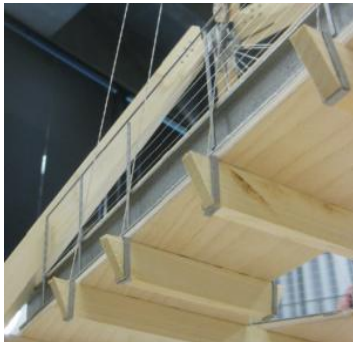
Fig. 4 Deck stringers cable support connection
