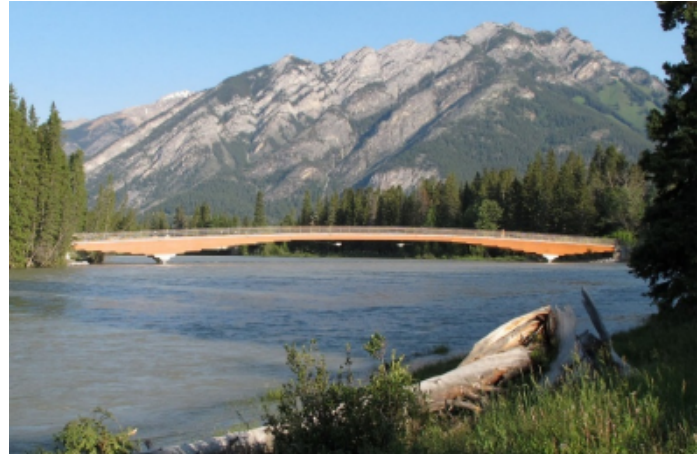
Figure 20 - Finished bridge south elevation
