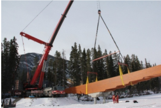
Figure 11 - Erection of south girders
