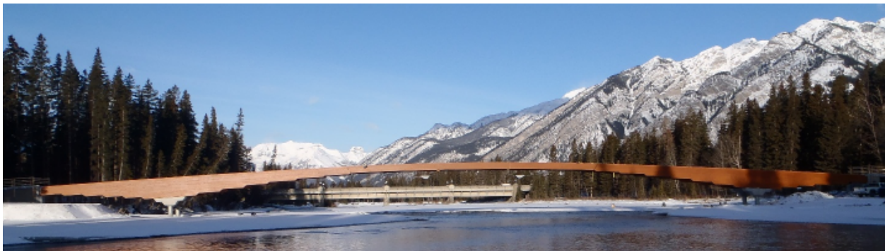
Figure 1 - Bridge superstructure after erection
