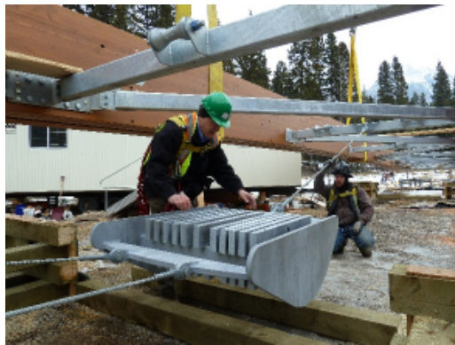
Figure 8 - Tuning of mass dampers before erection
