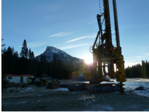
Figure 5 - Pile installation through the ice
