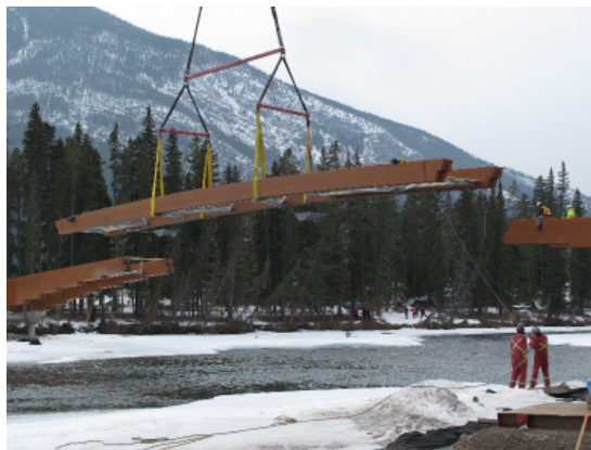
Figure 12 - Erection of drop-in span
