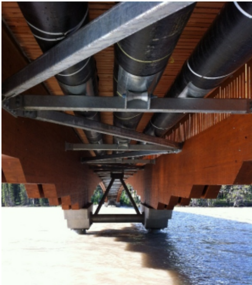
Figure 6 – Concealment of service pipes
