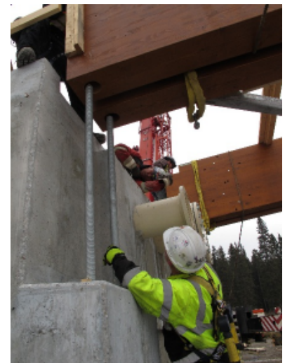
Figure 13 - Dropping over tie-down rods at abutment
