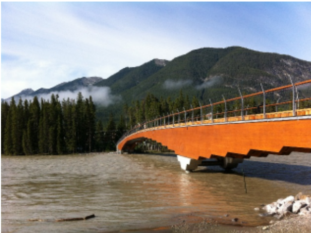
Figure 19 - Finished bridge south bank
