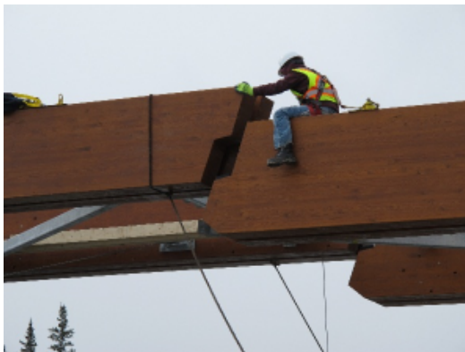
Figure 7 - Drop-in span detail
