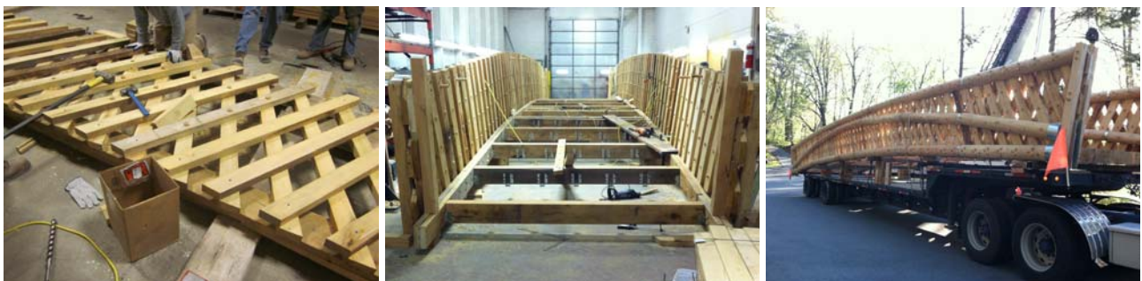
Fig. 7 TA Footbridge: truss layout, assembly, and delivery (photos by Tim Leiching).
