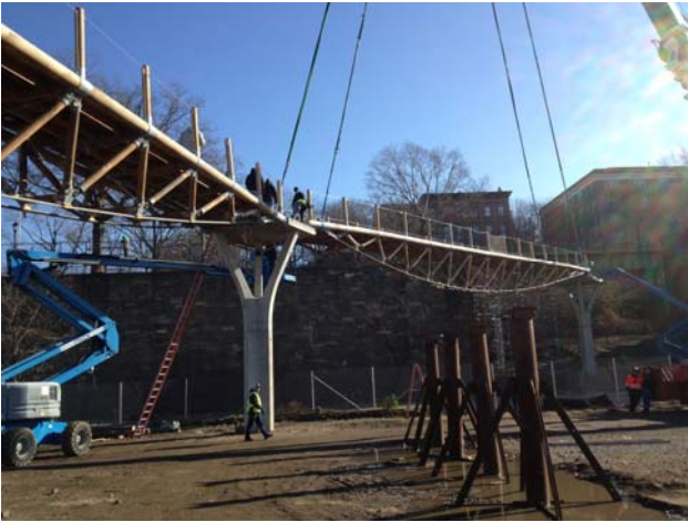
Fig. 1 Squibb Bridge: a) main spans assembled off alignment and erected with a single crane. Fig. 2 Squibb Bridge: exploded view.
