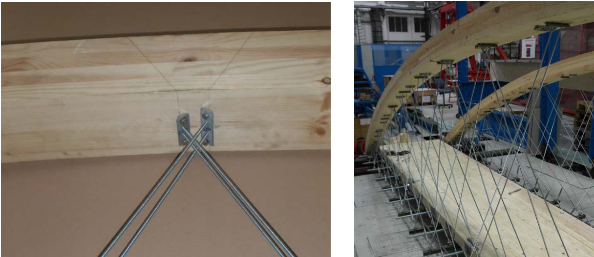
Fig. 13 Fastening of hangers to the wooden arch.
