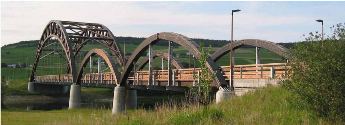
Fig. 1 Tynset bridge, Norway (photo: K. Bell)
