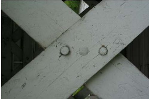
Existing bolted connection
