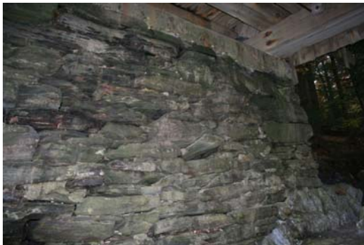
Field stone abutment
