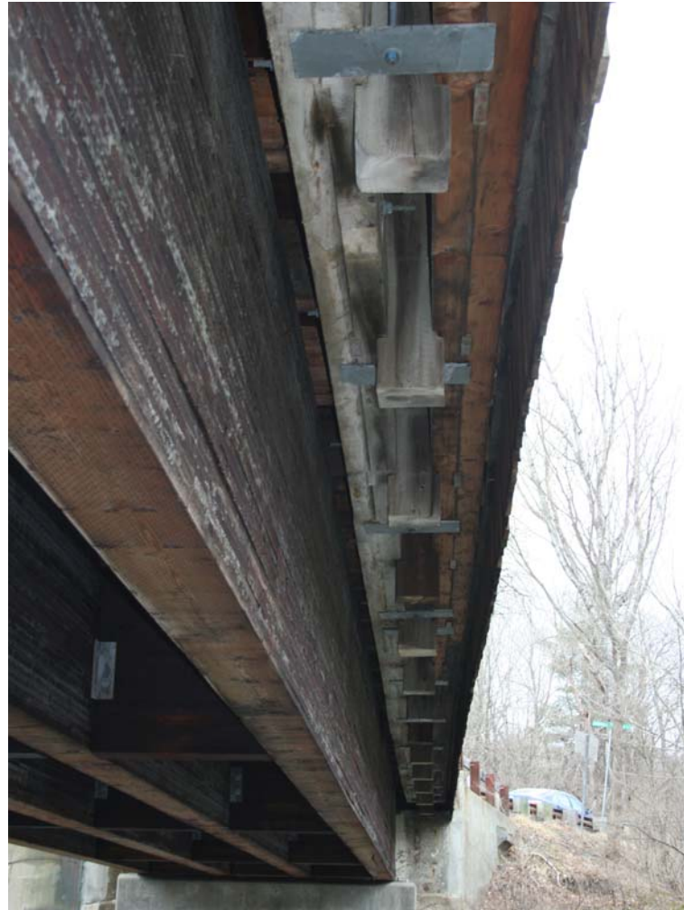
Co-functional glulam beams added
