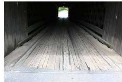
Sawn timber runners to hide glulam material
