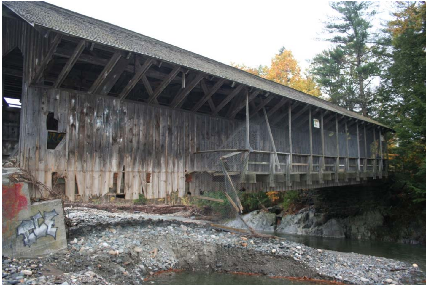
Green River Bridge Rehabilitation, Greenfield, MA
