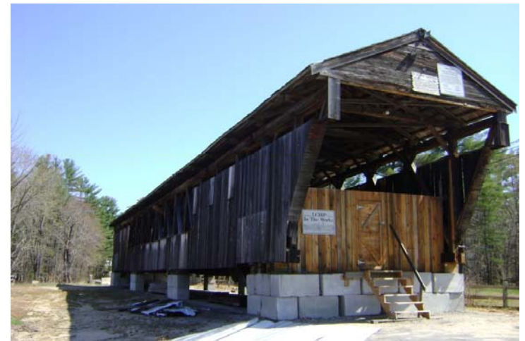
Whittier Bridge Rehabilitation, Ossipee, NH
