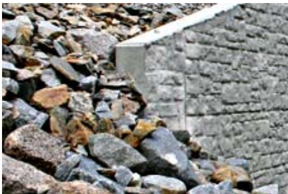
Stone pattern in concrete
