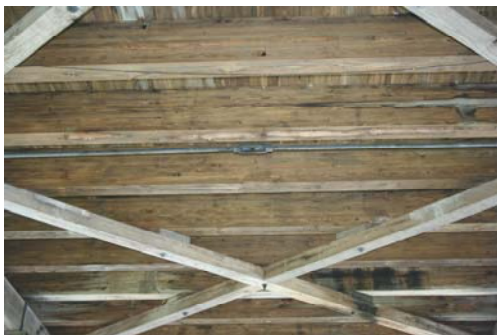
Glulam deck and floorbeams
