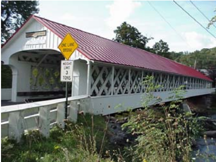
Bridge posted for 3-ton load
