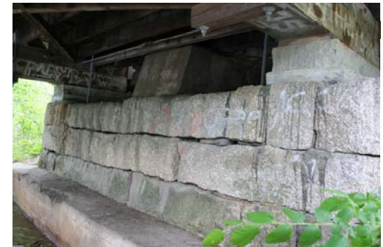
Granite block abutment
