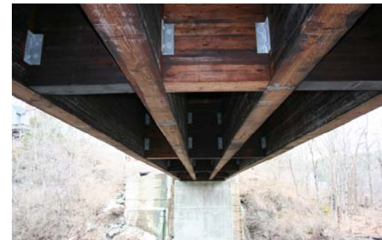
Glulam support system Union Village Bridge Thetford, VT
