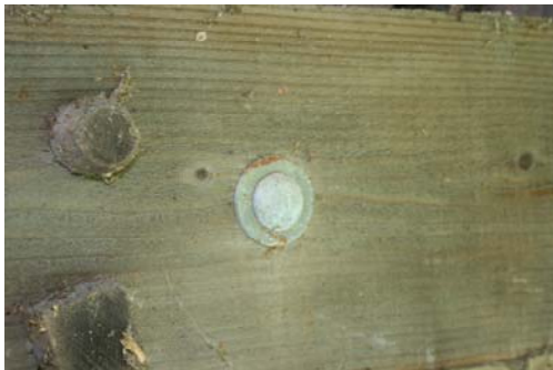
Standard carriage bolt with washer added
