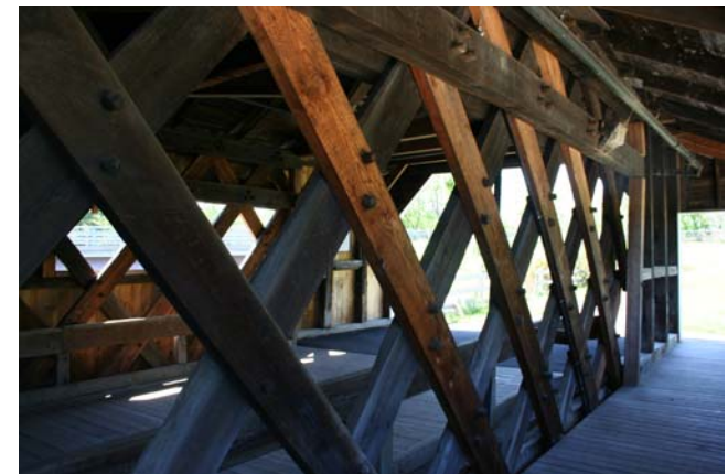
Web member strengthening Haverhill-Bath Bridge, NH
