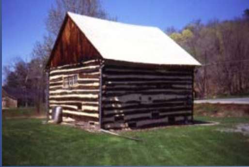
Log barn rehabilitation
