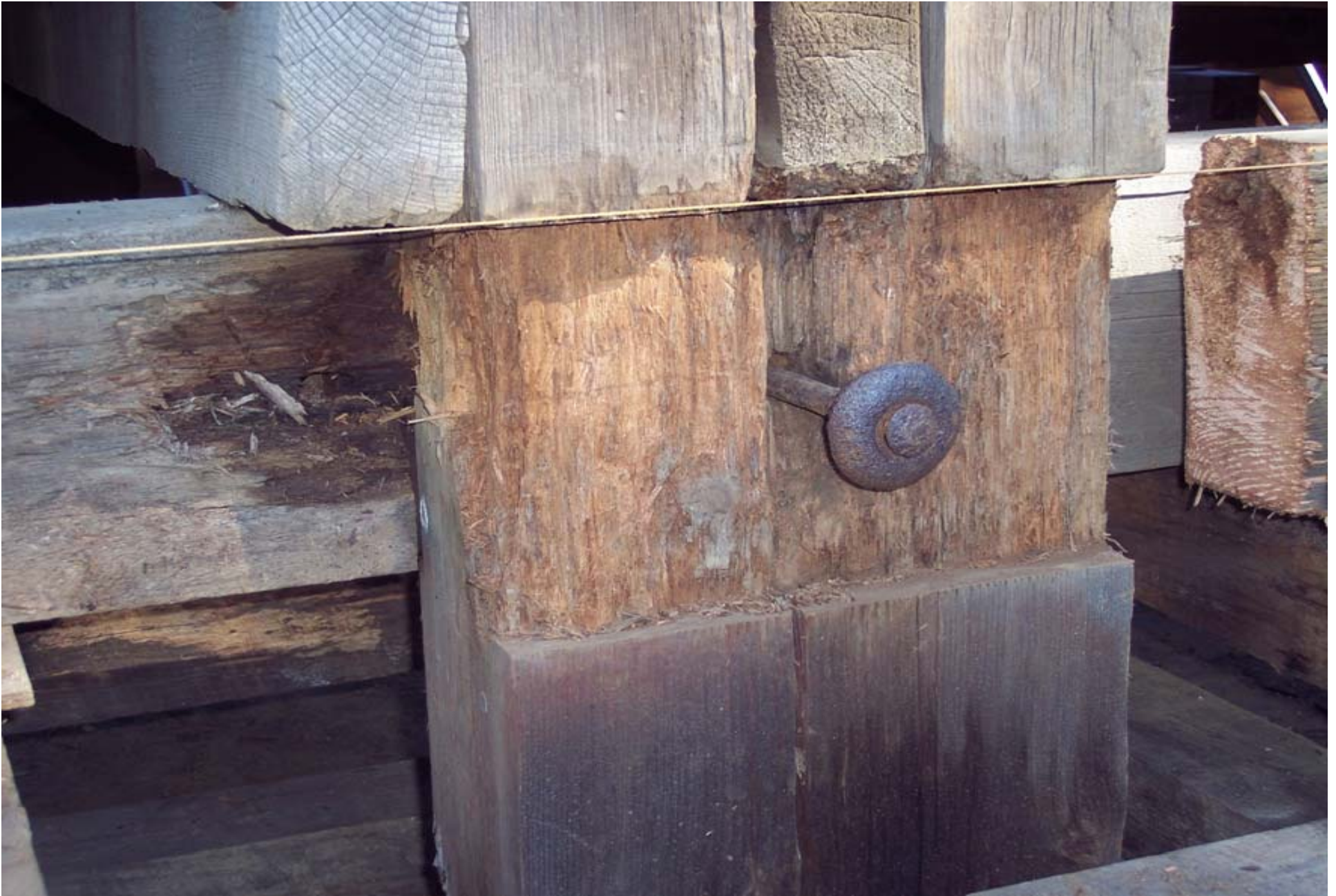
Floor beam framed through mid span king post
