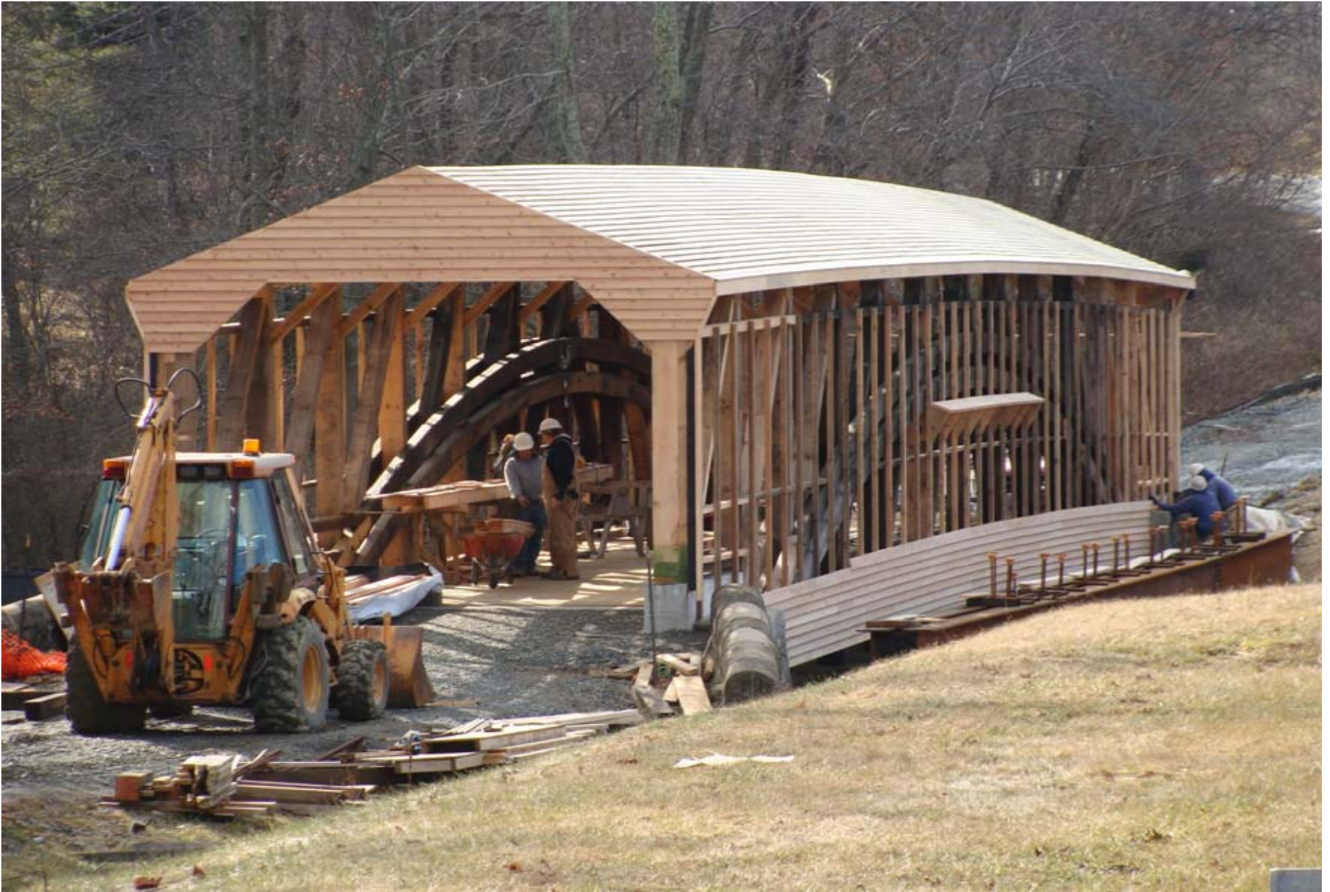
Close to completion
