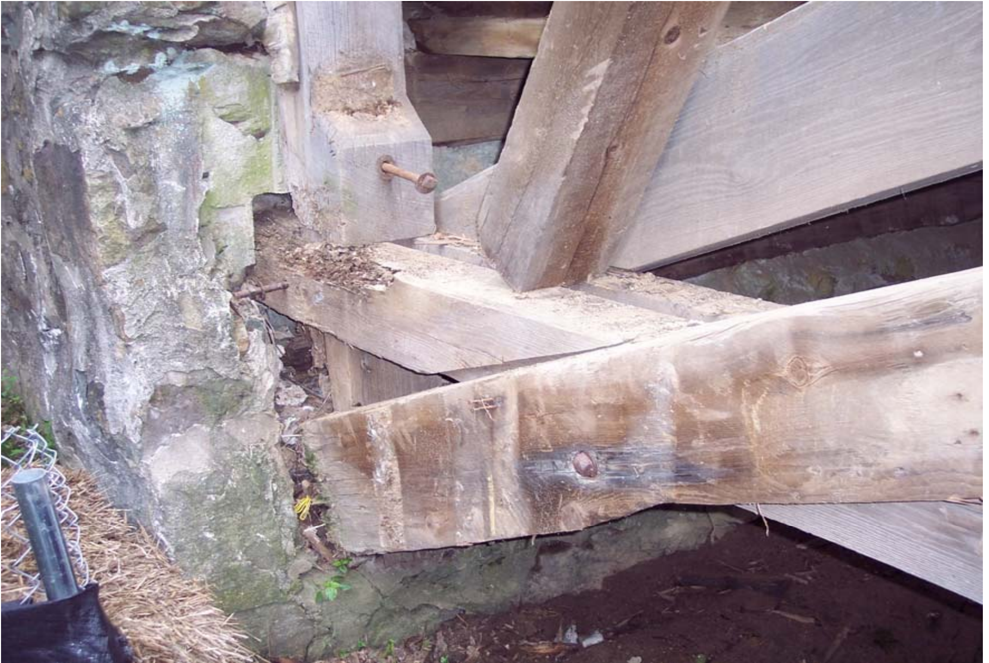
Embedded arch ends, bottom chord
