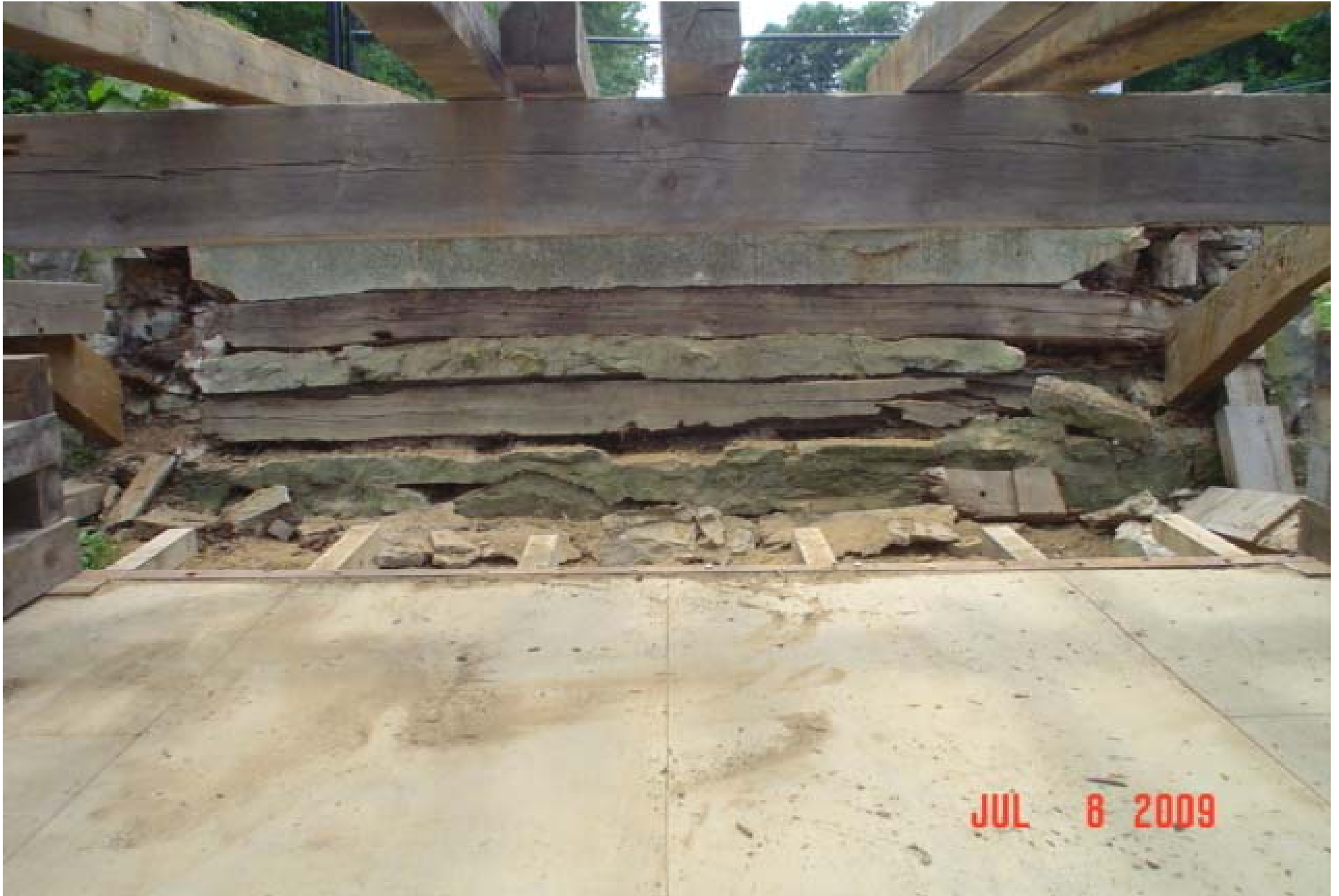
Embedded arch bearing timbers installed in 1959
