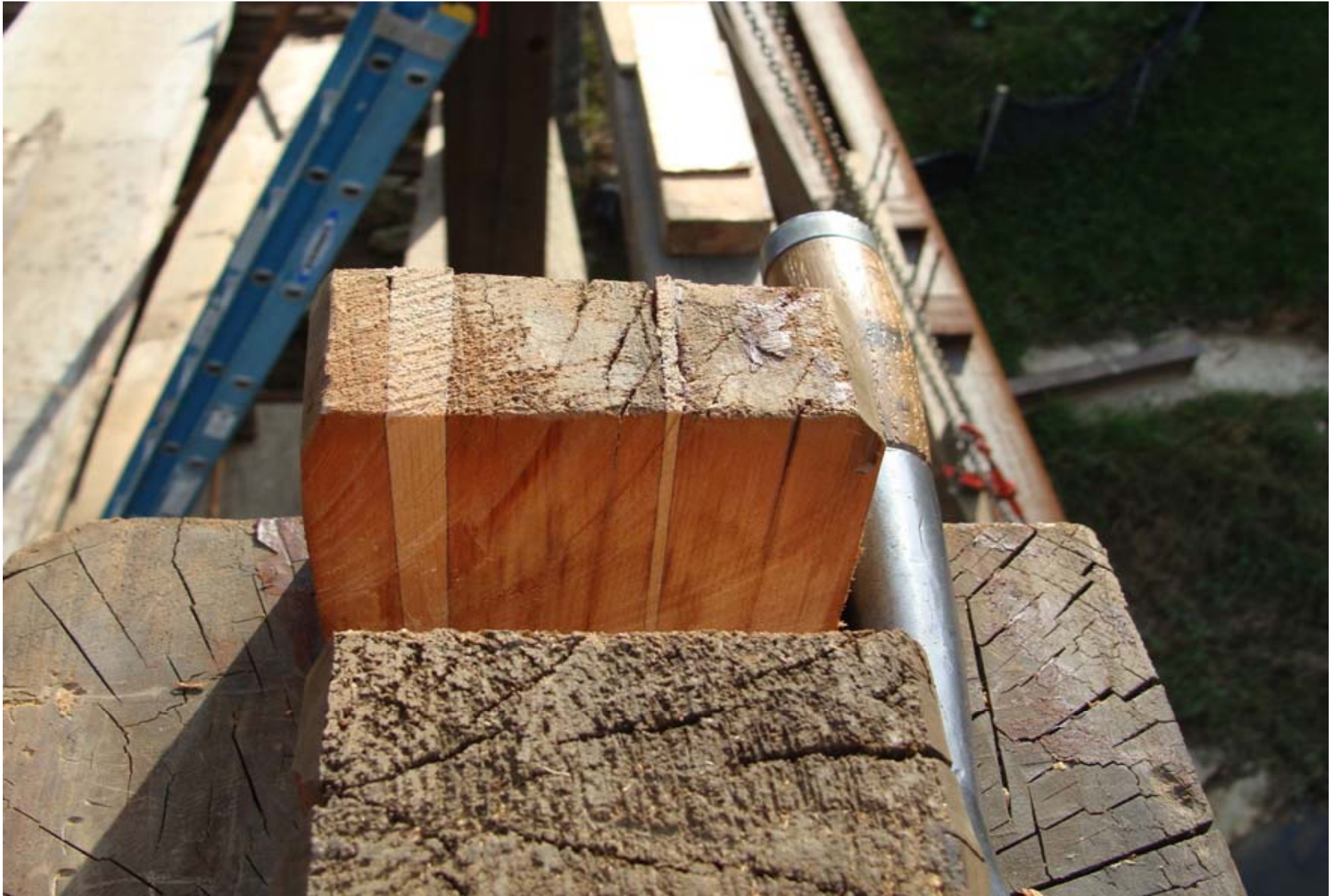
Prep for third glue up tight fitting Dutchman
