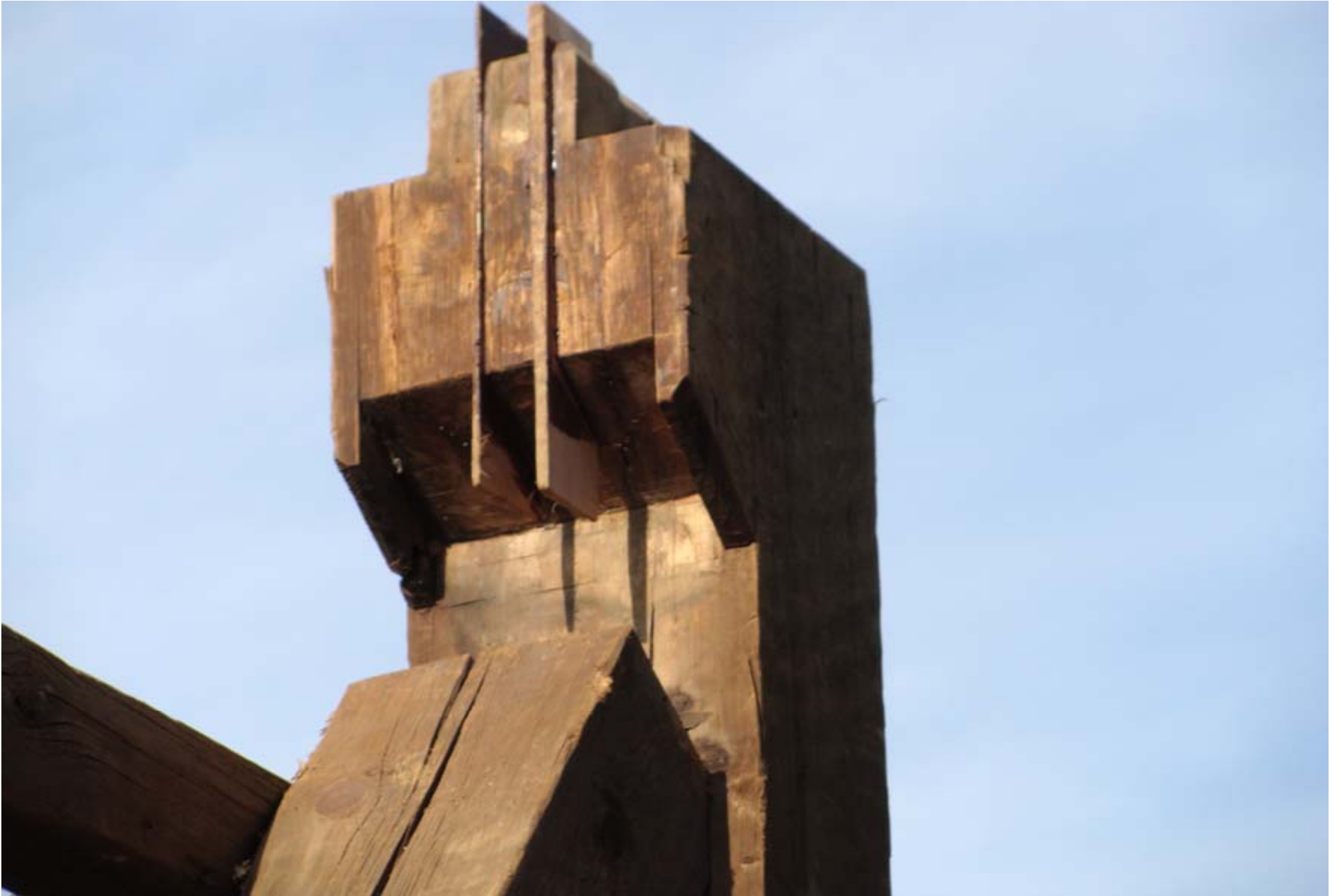
Second glue up of repair
