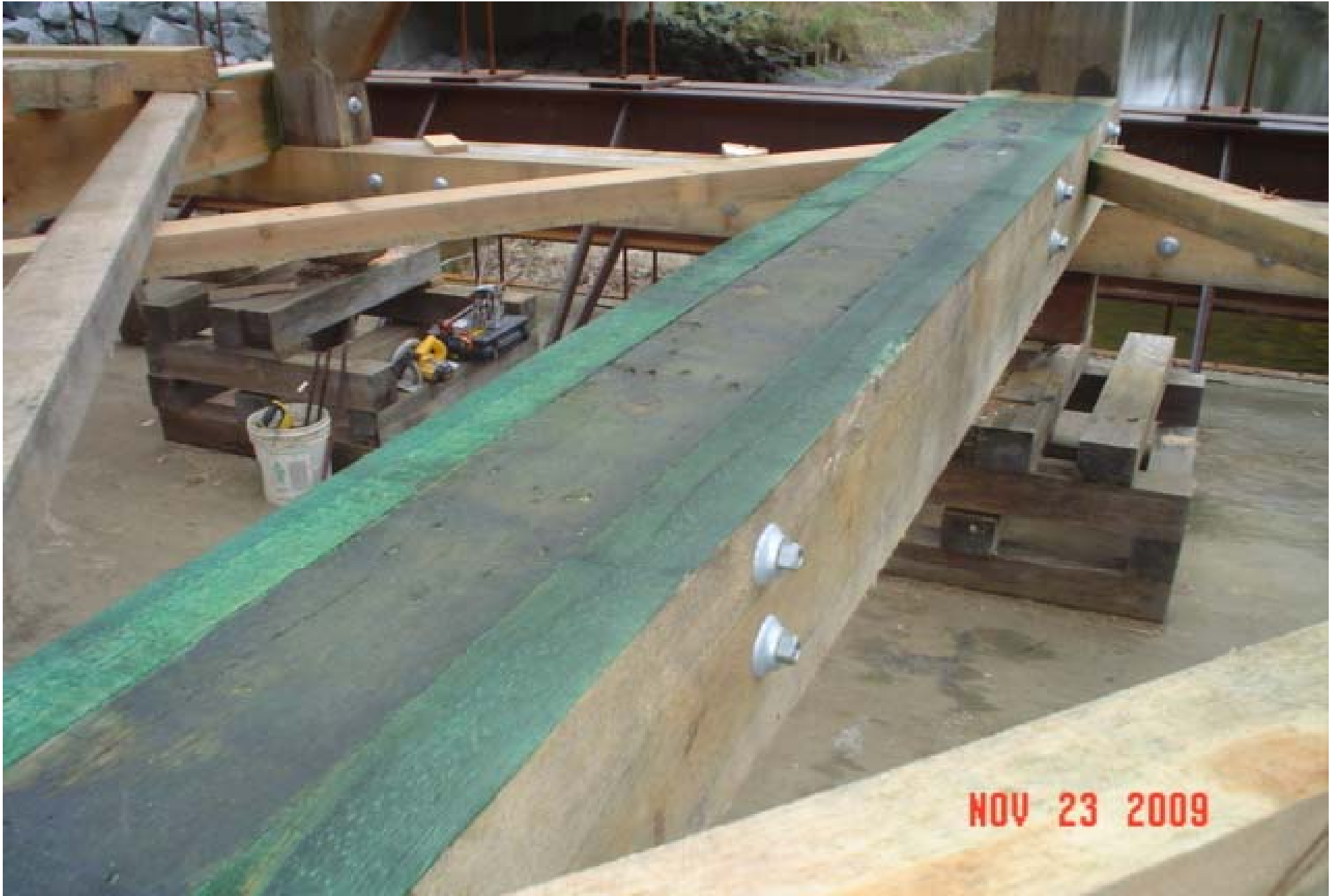
Original White Pine floor beam reinforced
