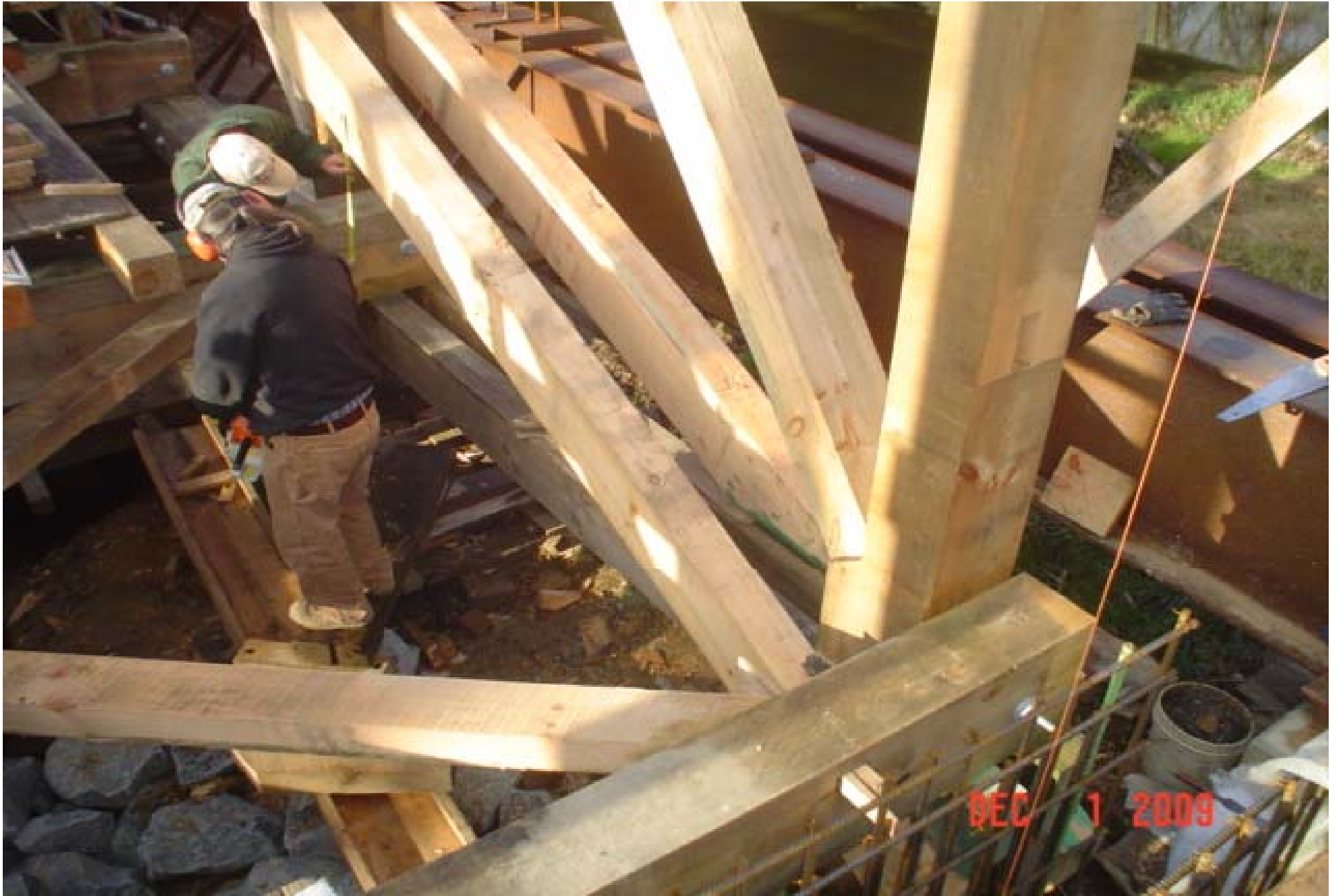
In kind replacements in materials and craftsmanship
