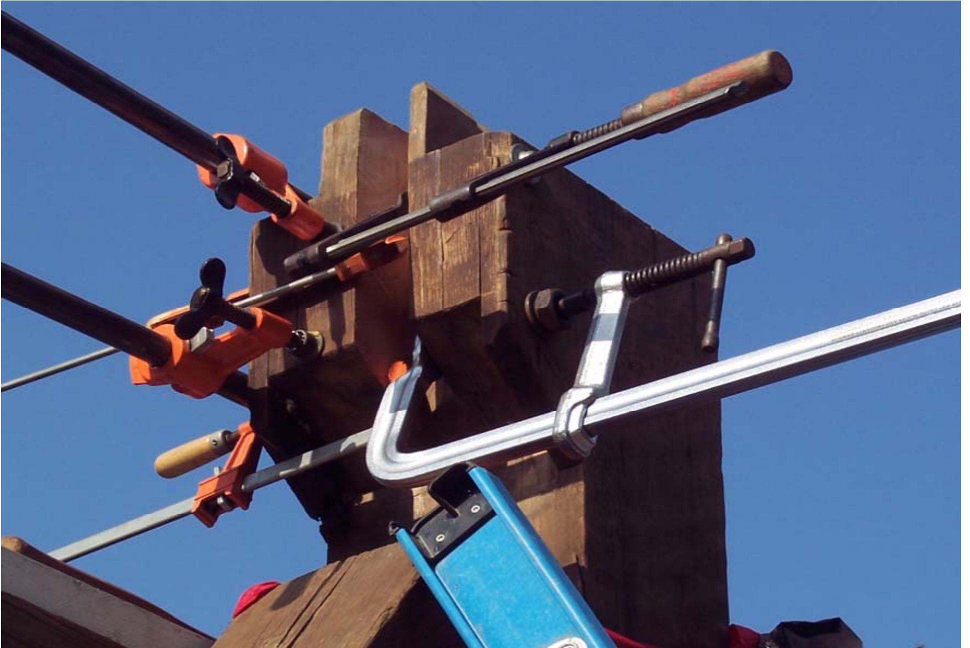
Initial glue repair
