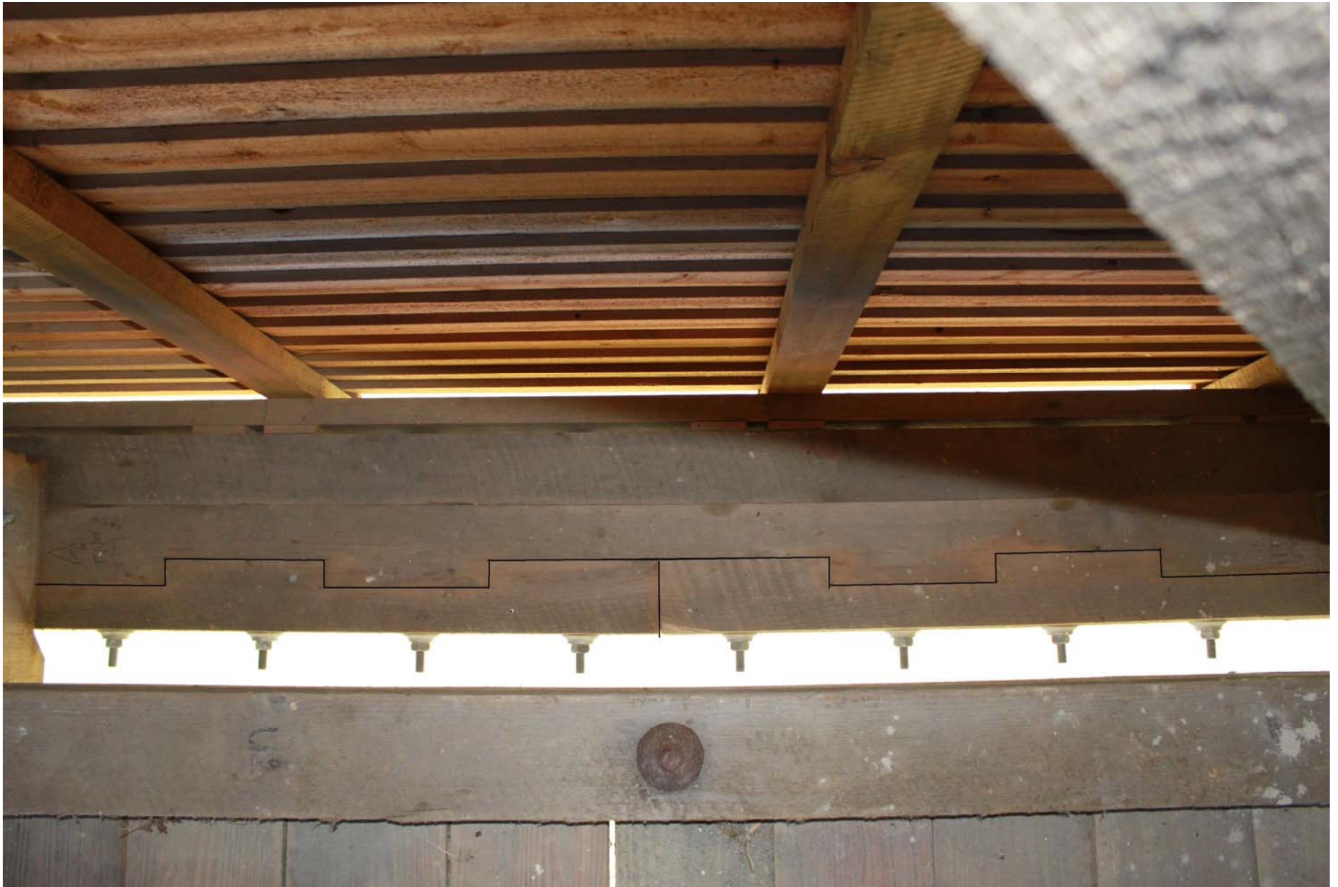
Modified shear connection
