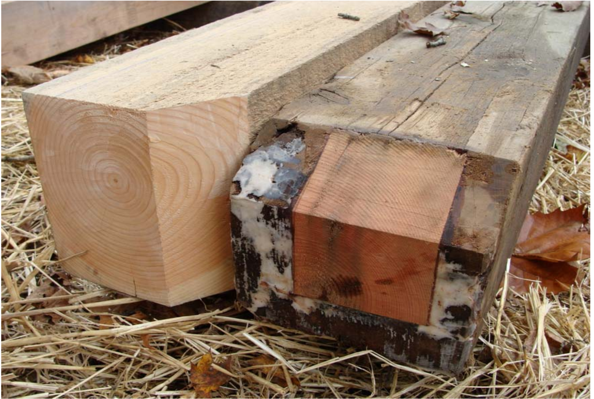
Hidden repair, epoxy used for shallow pockets
