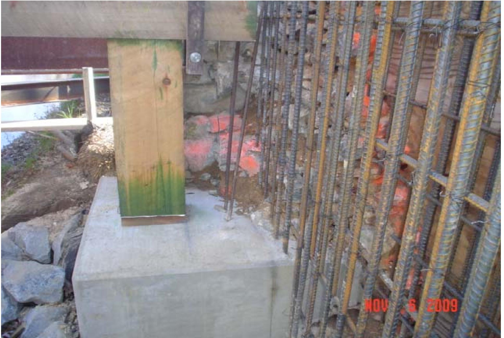
Design change- end posts atop concrete footings Black Locust spacers below
