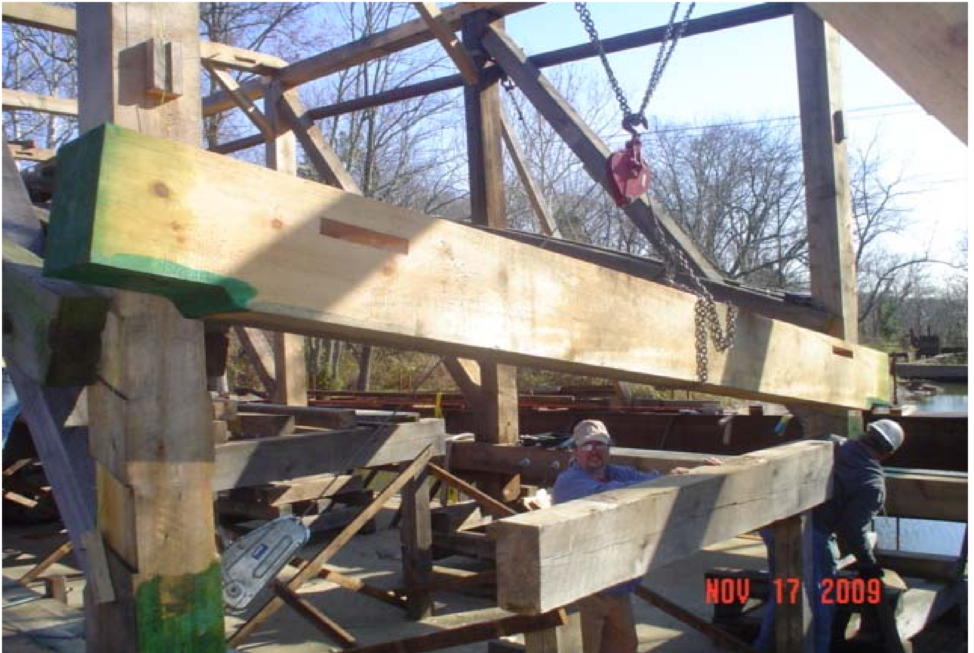
Replaced non historical Ash floor beam with historically correct White pine
