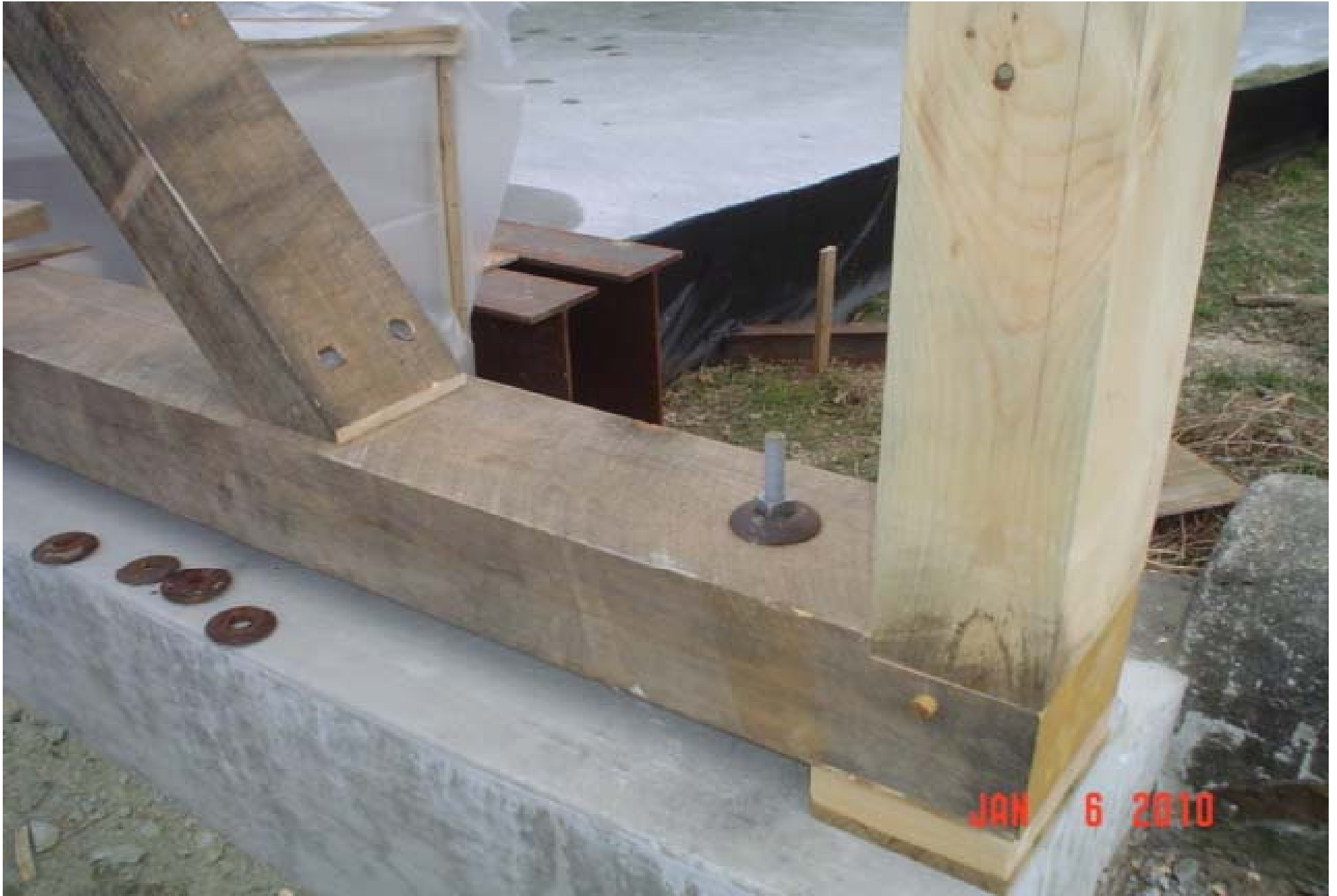
Restored shelter panel sill separated from concrete with Locust spacer
