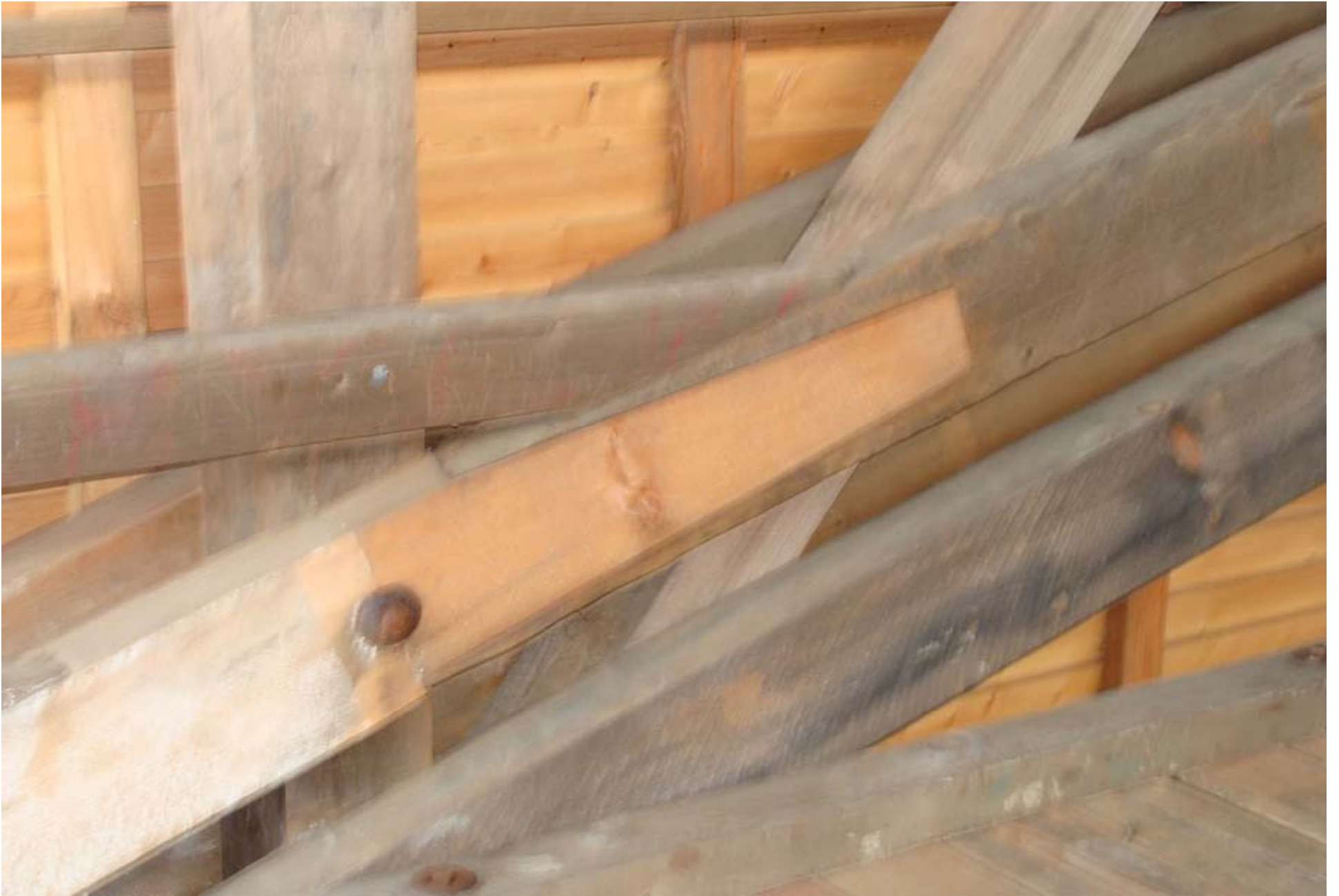
In line arch Dutchman repair
