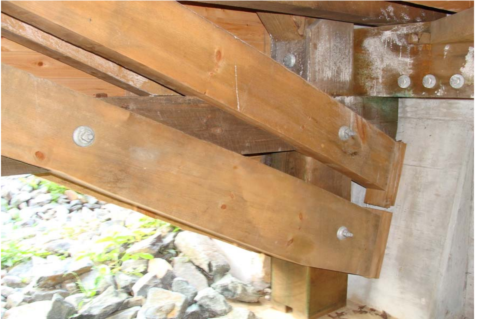
Locust wedges separate arch ends and post from concrete
