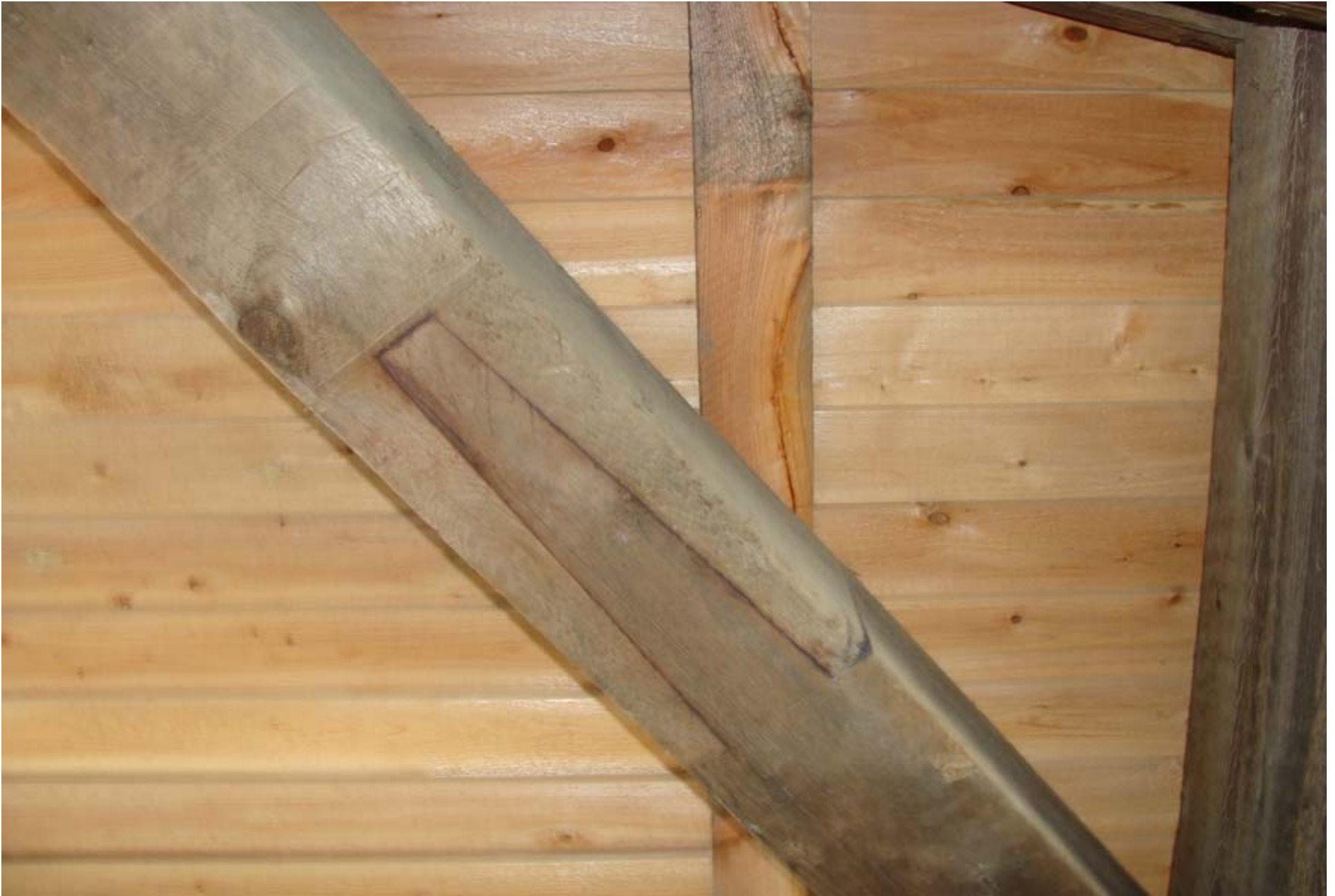
Clothespin scarf on truss brace
