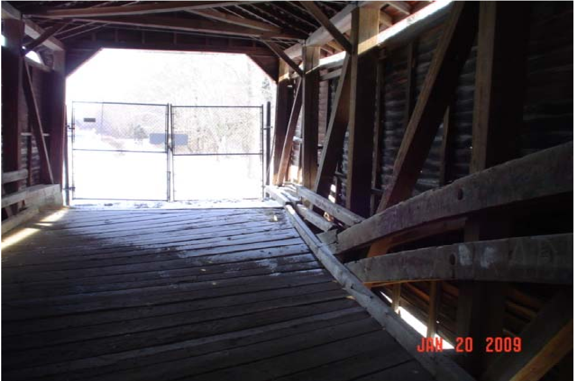
Pre construction floor plank arrangement
