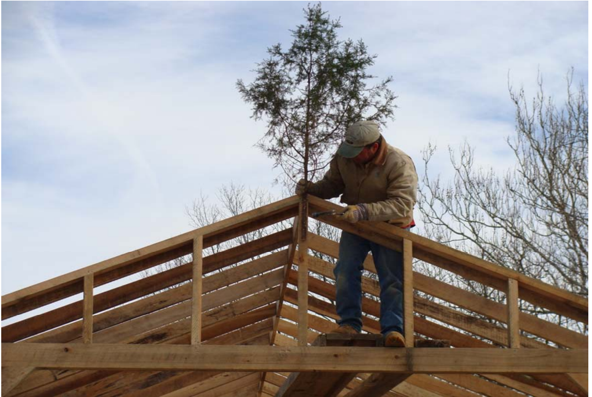
Preparing to “wet the bow” when last frame member in place
