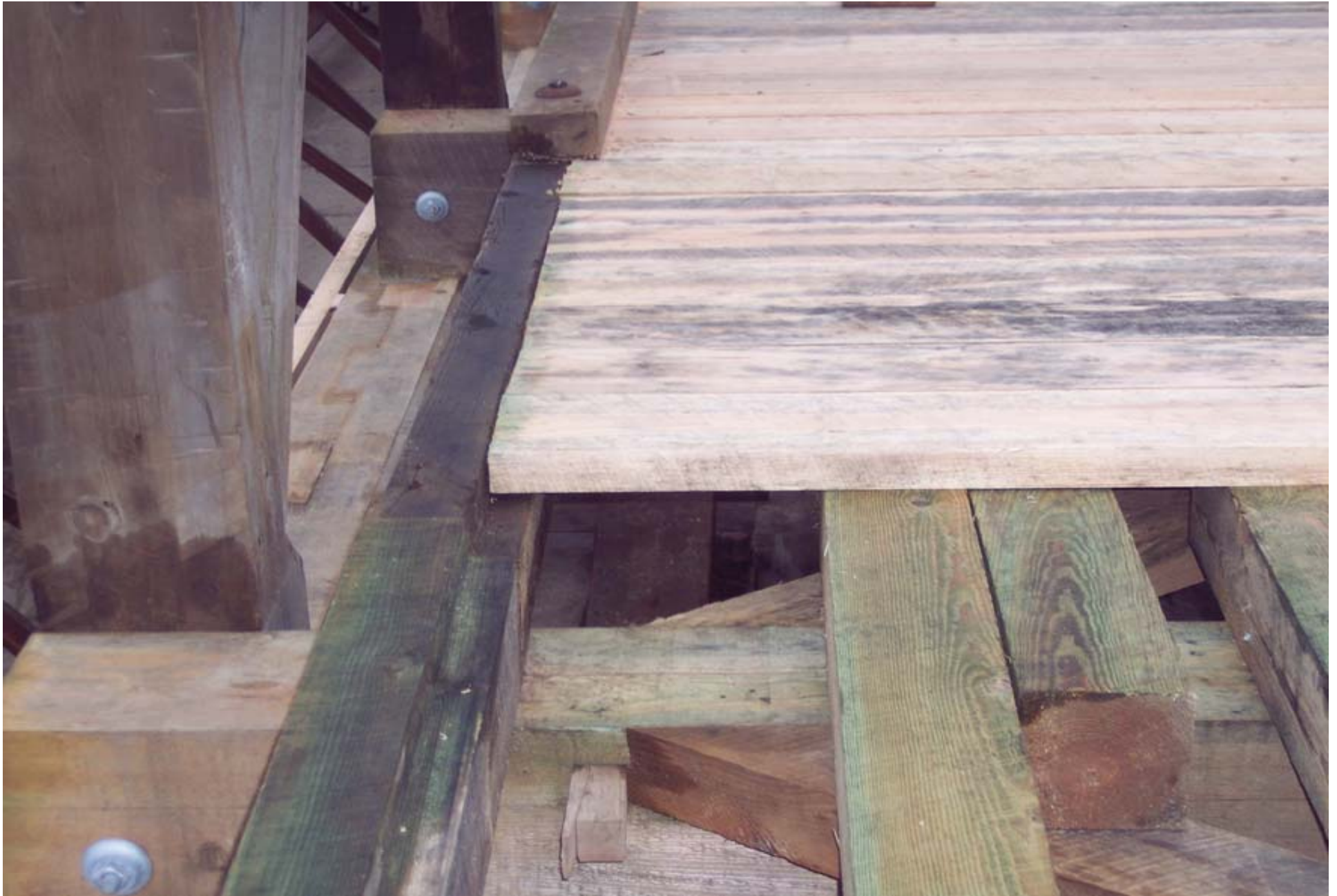
Nail free floor reproduced matching the original
