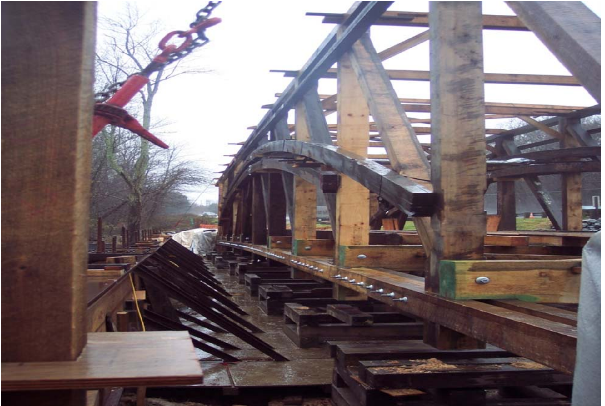
10" of camber restored, self supporting bridge
