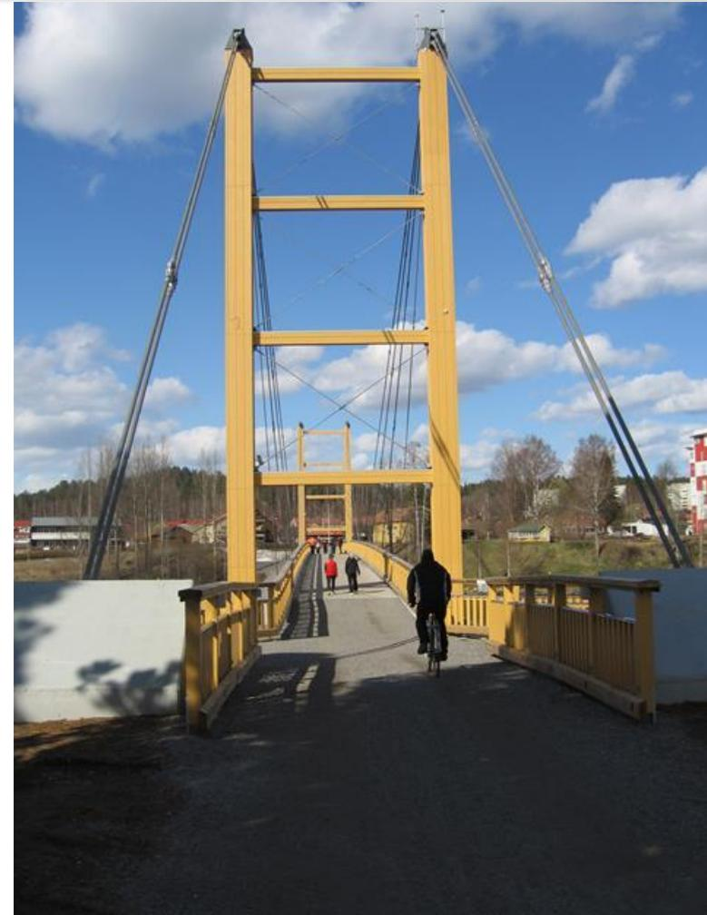
The total amount of glulam is almost 400 m<sup>3</sup> or 200 tonnes. There are also 80 tonnes of steel in the form of castings and fixtures of different kinds
