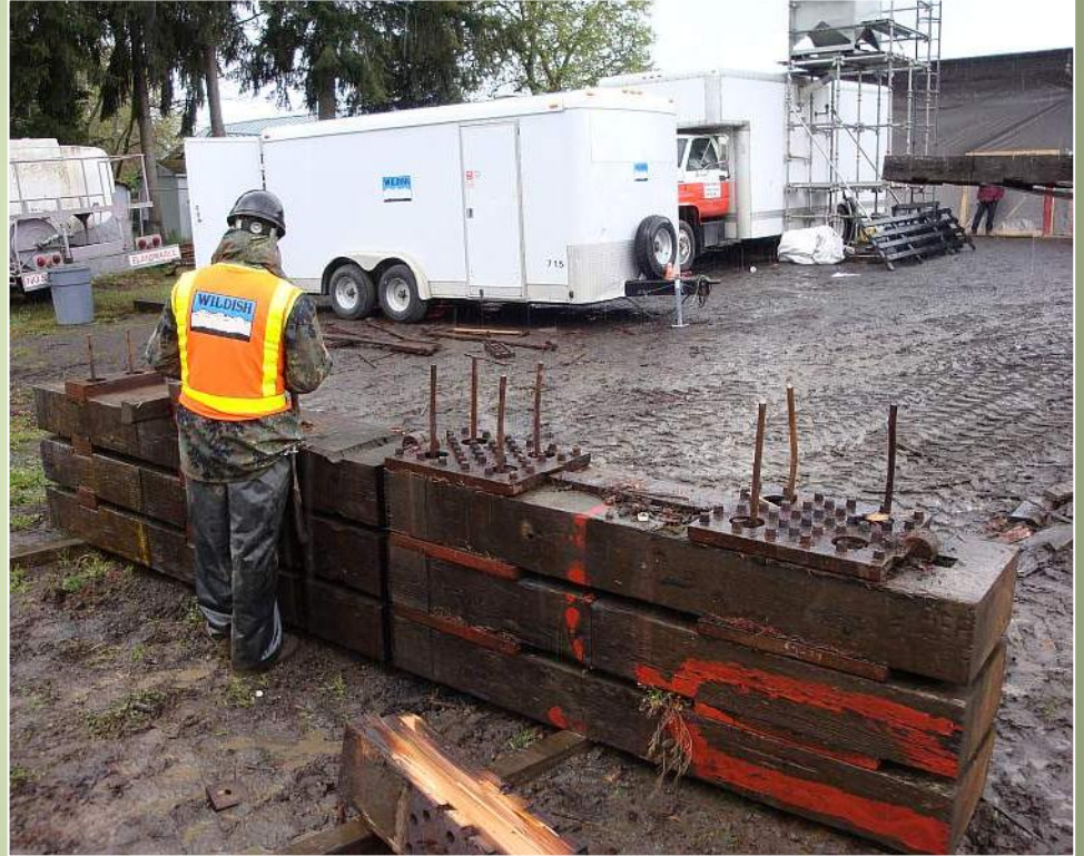
Splice assemblies kept together
