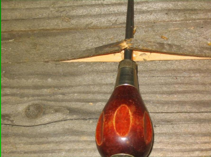
Decayed wood breaks abruptly across grain without splintering.
