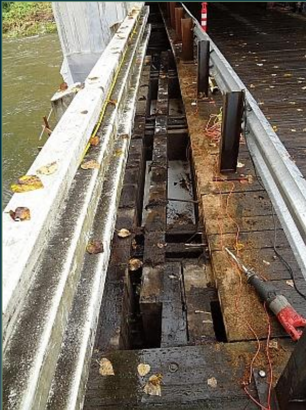
Temporary rail installed and deck cut
