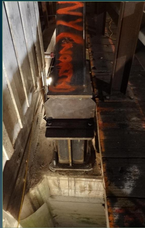
Bearing on concrete pier
