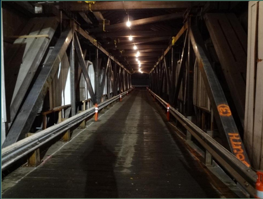
Ready to lift timber bridge
