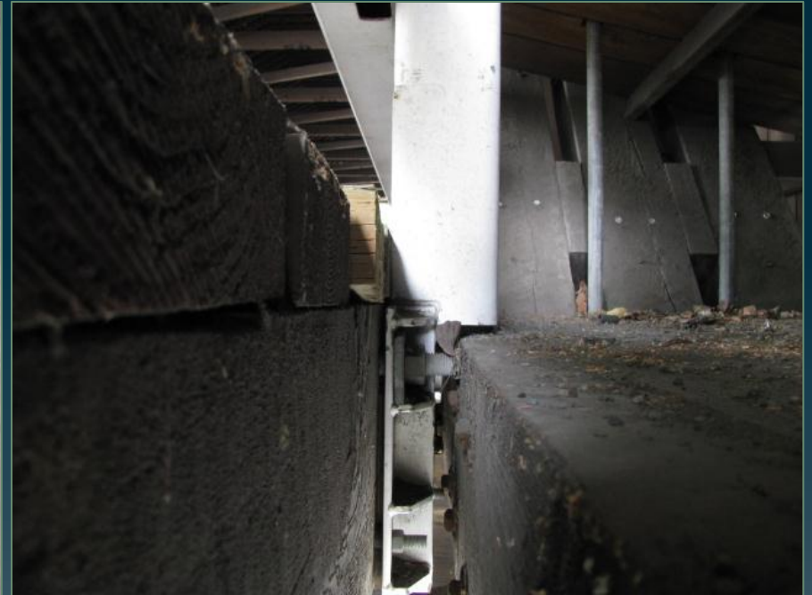
Between rail post and bottom chord
