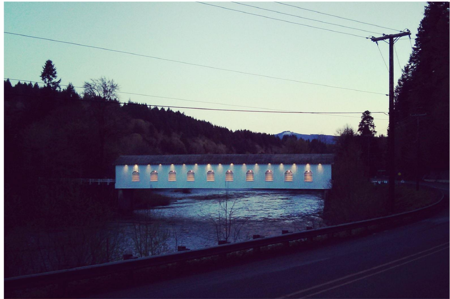
GOODPASTURE COVERED BRIDGE, 2013
