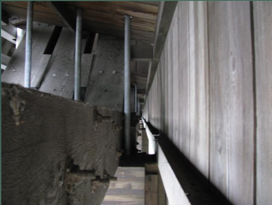
Between bottom chord and siding
