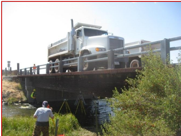
Upper Williamson bridge
