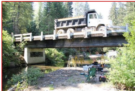
Lost Creek No.2 bridge
