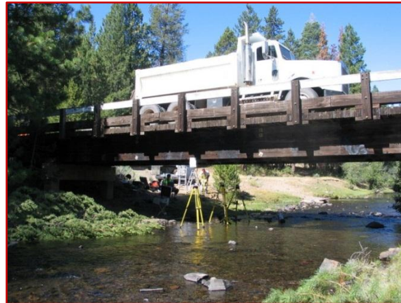
Elder Creek bridge
