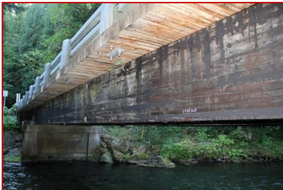
Panther Creek bridge
