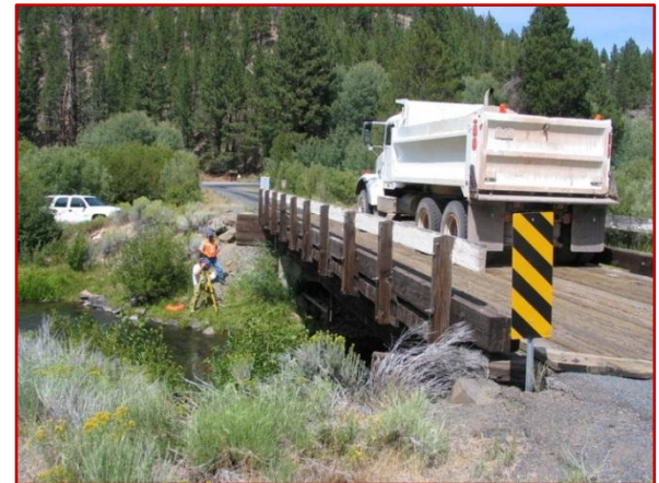
Dairy Creek bridge
