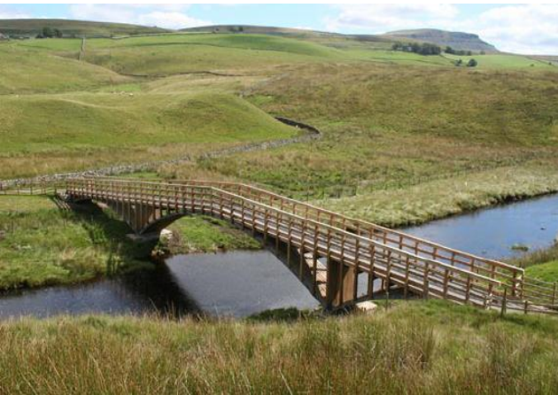
Case Study 5 Far Moor Bridge Yorkshire, UK Stress-Laminated Arch
