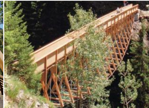
Case Study 4 Travesina Bridge Viamala, Switzerland Truss
