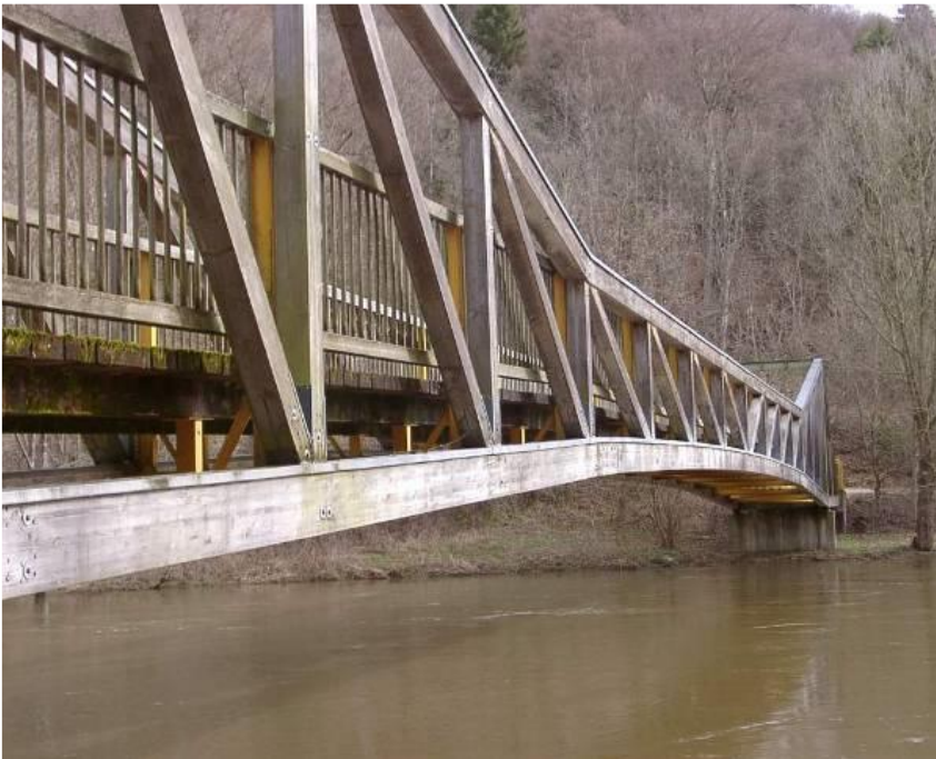
Pedestrian and bicycle bridge over Danube near Dietfurt
