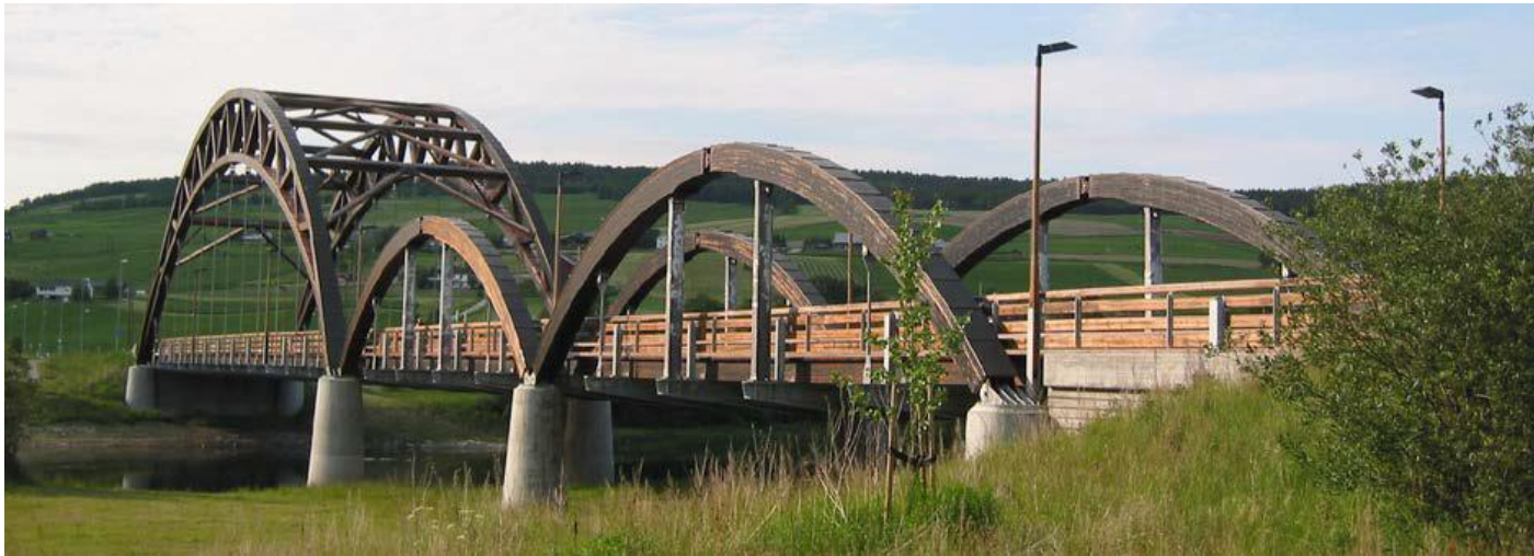
Tynset bridge, Norway (photo: K. Bell)
