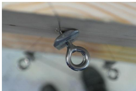
Fastening of hangers to the wooden arch
