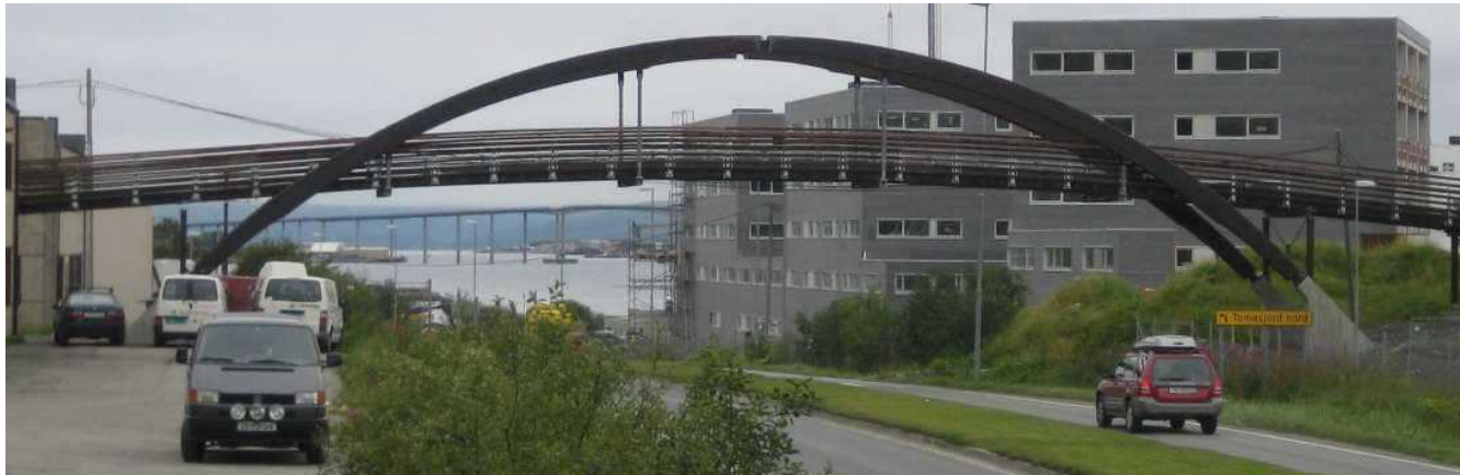
Footbridge, Trømso, Norway (photo: SWECO)
