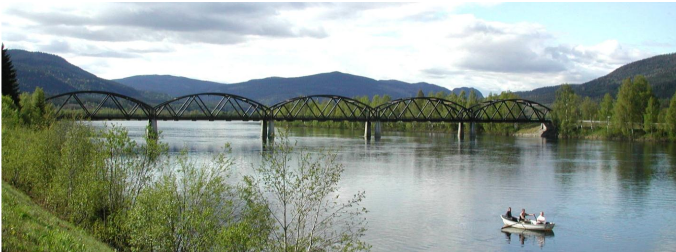
Evenstad Bridge 5 span, 180 m long, constructed in 1995
