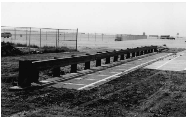
FIGURE 1 Bridge railings successfully crash tested to AASHTO PL-1 (longitudinal deck).
