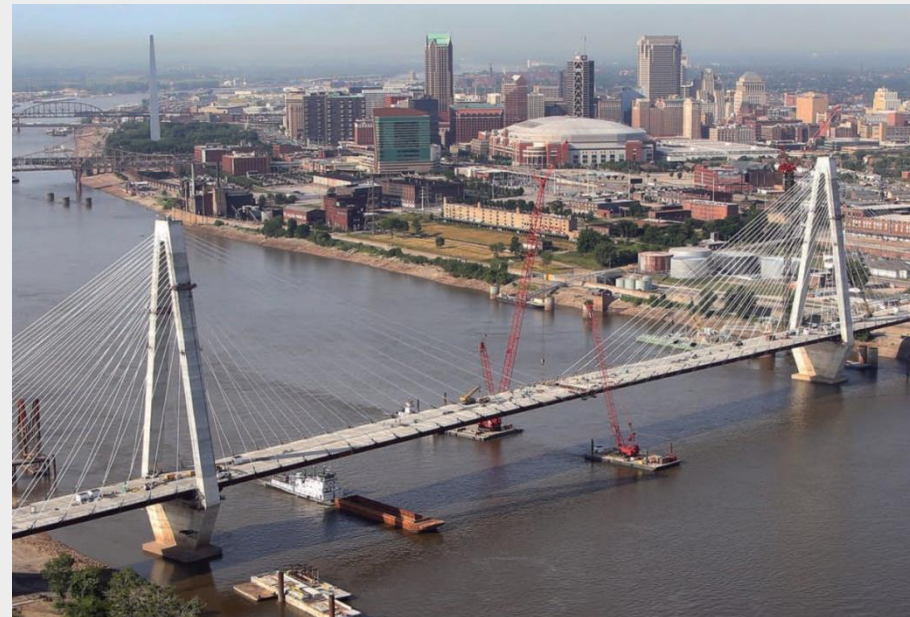
I-70 Mississippi River Bridge, St. Louis
