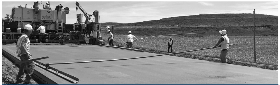
Hand finishing (The Transtec Group, Inc.)
