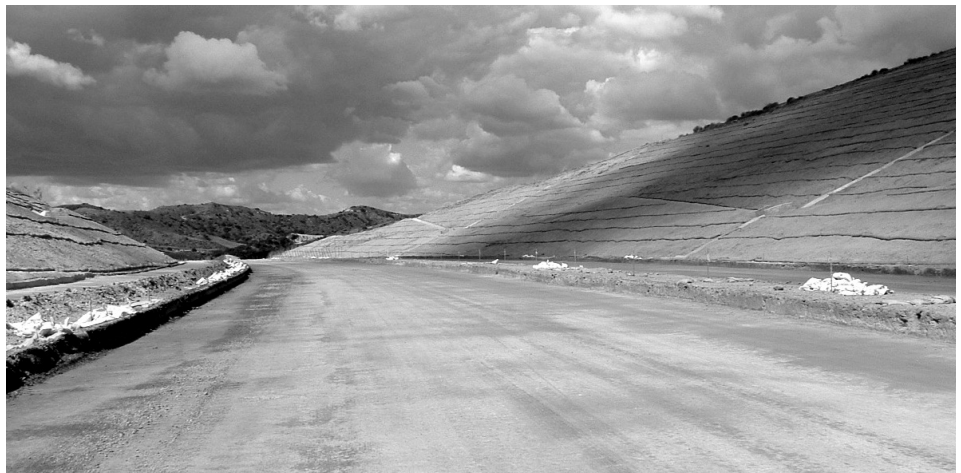
Compacted subgrade (Jeff Wykoff, California Nevada Cement Association)
