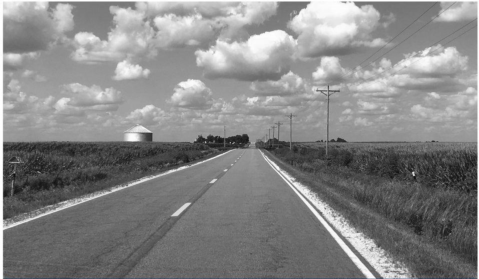
Microsurfaced pavement in Hamilton County, Iowa
