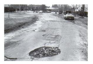
1. Pothole caused by fatigue failure.
