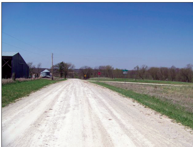
Looking at Y intersection along one leg
