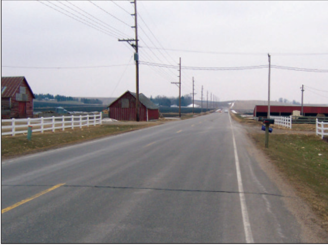
Photos show additional paved foot for errant vehicles (photos courtesy of Bob Sperry)
