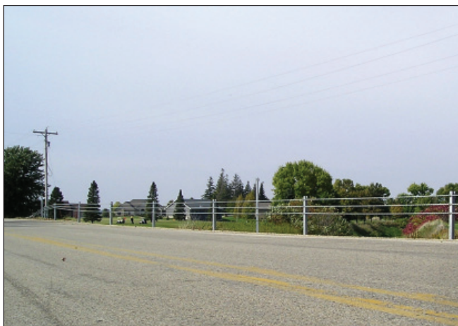
Cable guardrail for embankment area (left) and at curve location (right) (photos courtesy of Tom McDonald)
