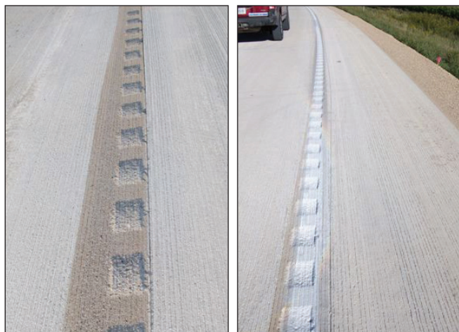
After milling (left) and with paint applied (right) (photos courtesy of Linn County)
