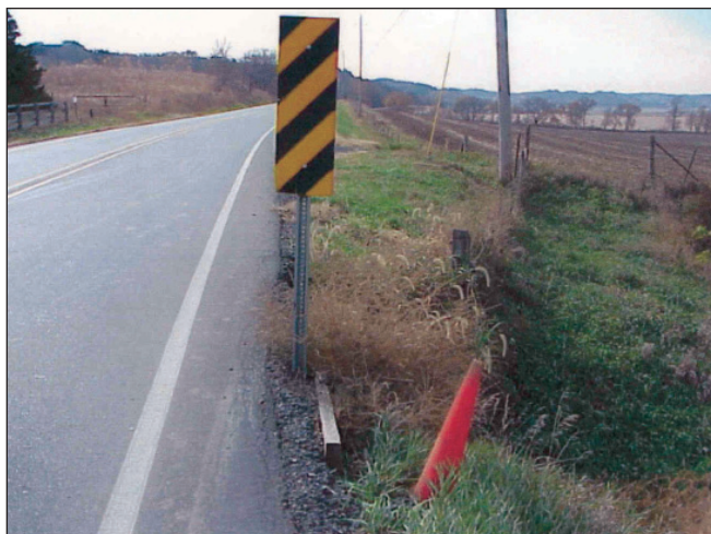
Object markers at culvert hazards (photos courtesy of Bob Sperry)
