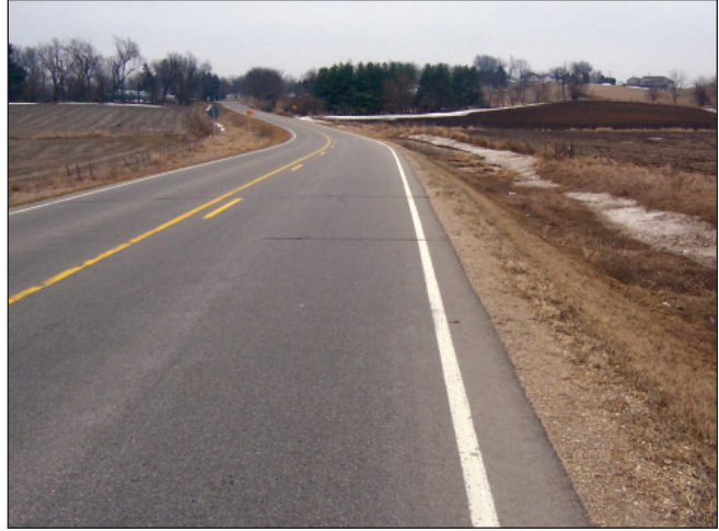
Photos show additional paved foot for errant vehicles (photos courtesy of Bob Sperry)
