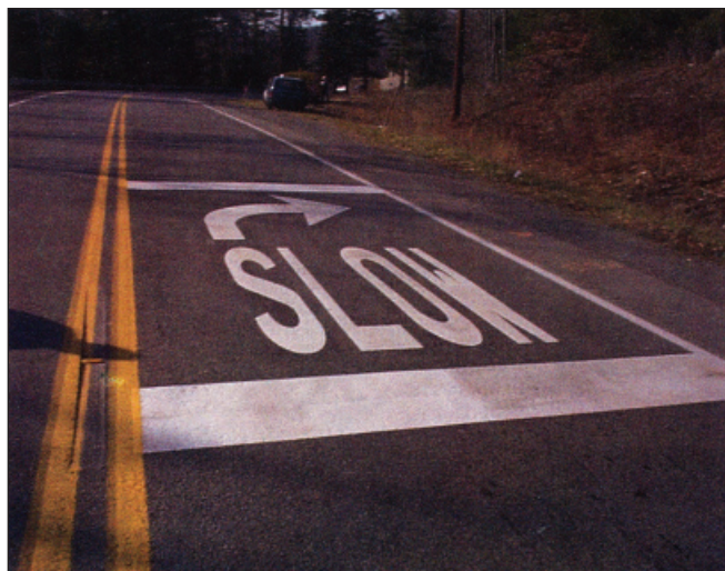
PennDOT curve advance marking (photos courtesy of Federal Highway Administration)
