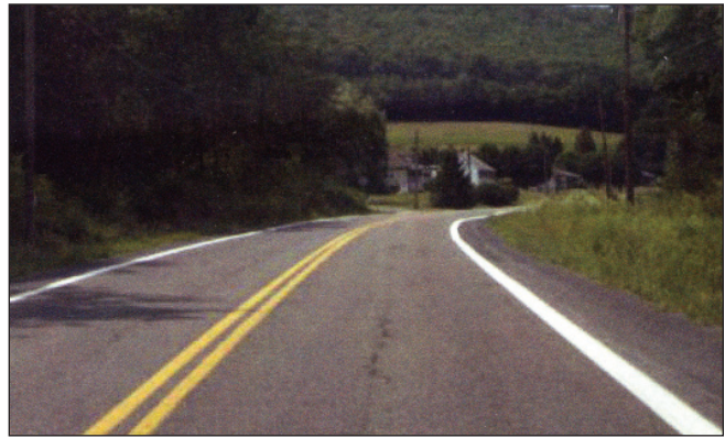
Roadway with 8 in. edge line
