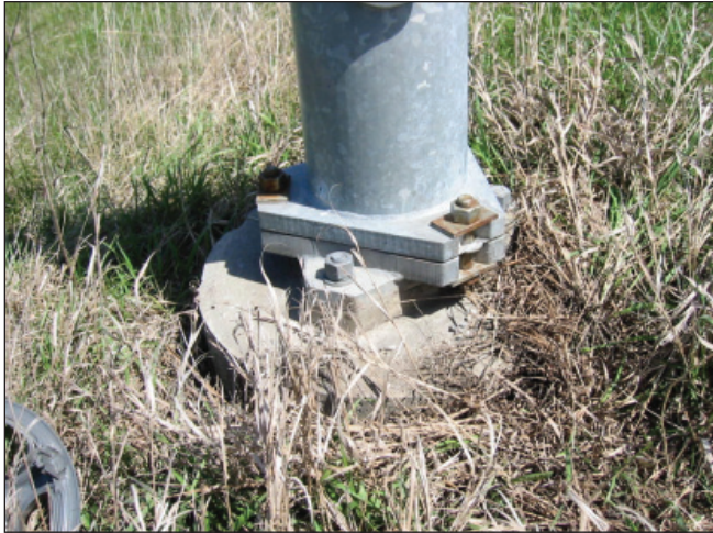
Breakaway base closeup (photo courtesy of Iowa DOT)
