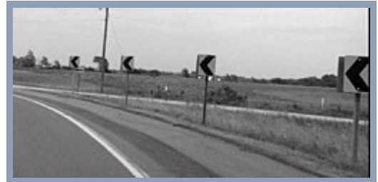
Bigger and brighter chevrons and rumble strips protect drivers from running off the curve on U.S. Highway 69 in Clarke County.
