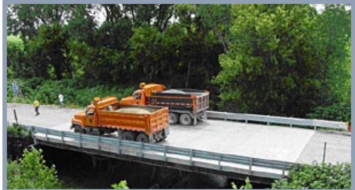
Above are two other Tama County modified beam-in-slab demonstration bridges.
