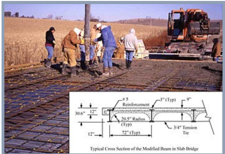
Tama County bridge under construction. Inset: Typical cross-section of the modified beam-in-slab bridge.
