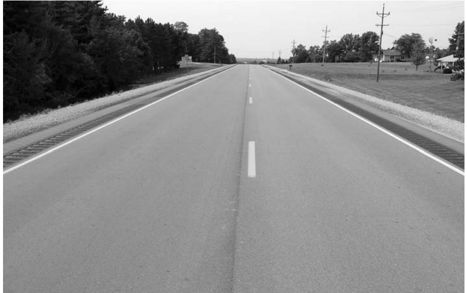
A two-lane Iowa highway with shoulder rumble strips. (Photo courtesy of Jack Latterell)
