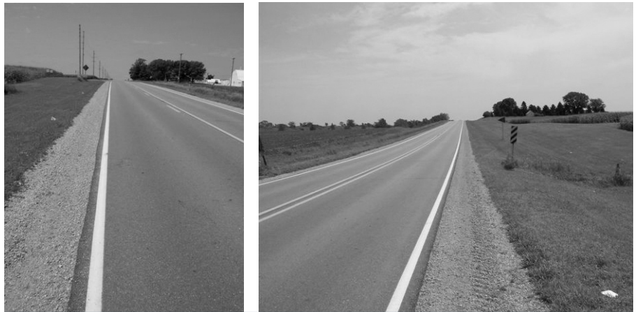
Two-lane roads with recently painted edgelines. (Photos courtesy of Bob Sperry)
