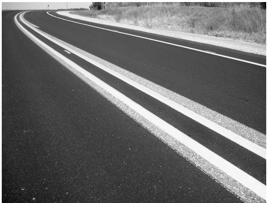
A milled in centerline pavement marking. (Photo courtesy of Tom McDonald)
