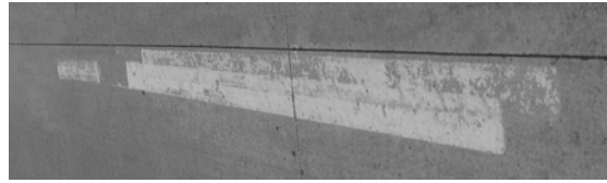
Water-based paint markings (above) are typically replaced every six months to two years.
