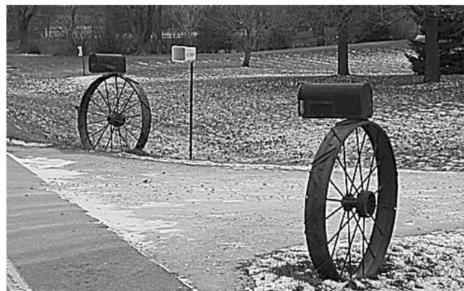
Some mailbox supports in the right-of-way can be dangerous for errant vehicles.
