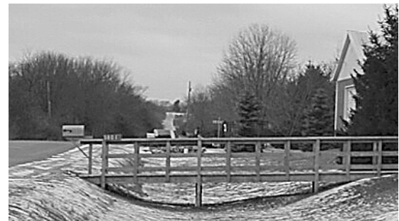
Other right-of-way obstructions (top to bottom): driveway retaining walls, crops, and footbridges
