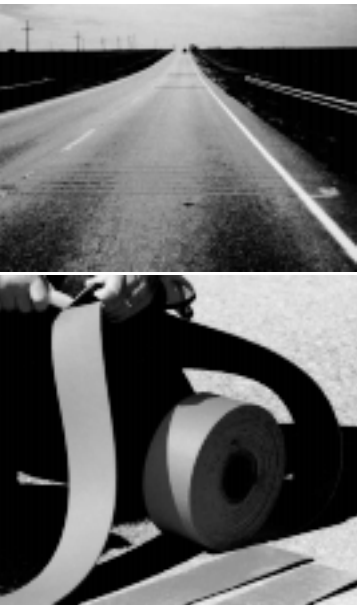
Removable orange rumble strips warn drivers approaching a work zone.
