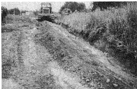
Above, a typical muddy, rutted road in rural Russia near St. Petersburg. Below, Alvin Jansen widens the road and builds the crown.
