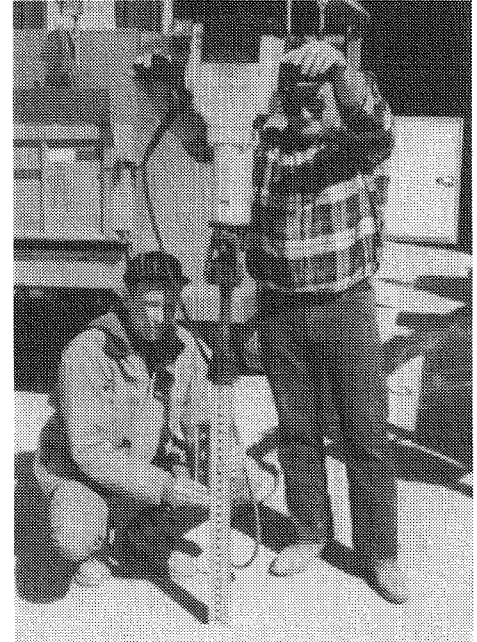
Muscatine County signmen Doug Holiday (left) and Wayne Martin show how they install the ground section of the square steel post system.
