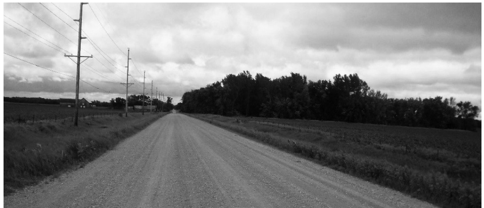
Figure 1. Straight, level, “hazard free” roadway in Story County
