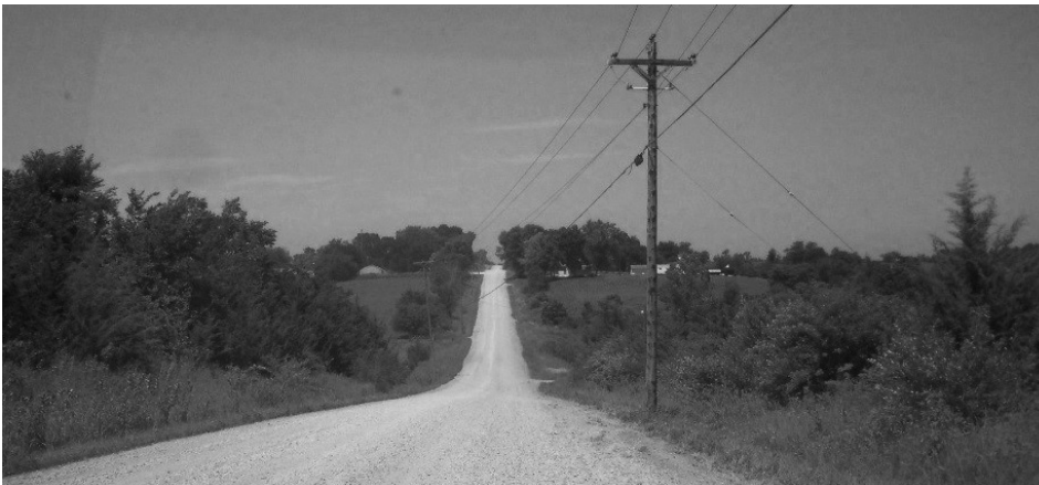
Figure 2. Utility pole located very close to the road shoulder, well within the clear zone, is a safety hazard
