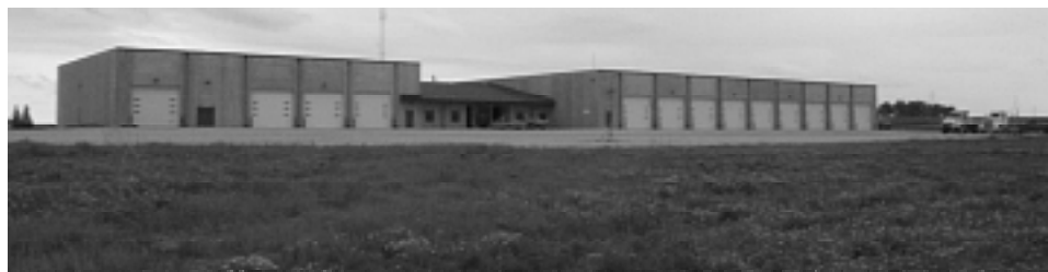
This new maintenance facility is a joint project of Floyd County, Charles City, and the Iowa DOT.
