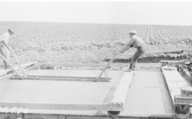
Workers using an early concrete pavement finisher, circa 1920s. Photo courtesy of Iowa Concrete Paving Association.
