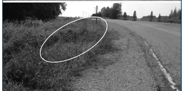
Cable guardrails at an embankment area (top) and at a curve location (bottom). (Photos courtesy of Tom McDonald)
