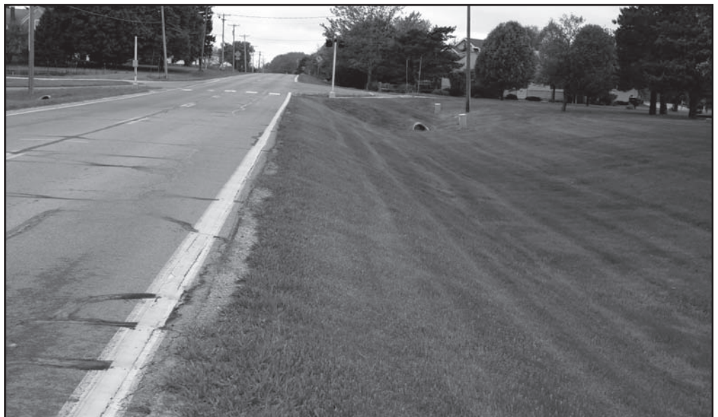
An example of a ditch with good drainage.
