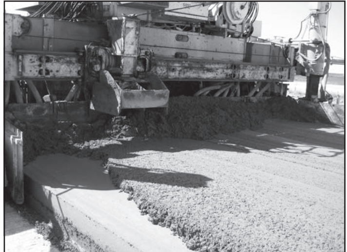
Two-lift paving involves the placement of two wet-on-wet layers of concrete.
