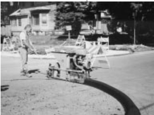
This temporary asphalt curb was installed during the summer of 1998. It has since been replaced with a permanent concrete curb.
