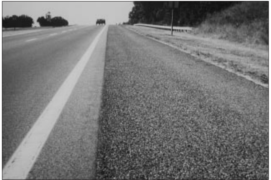
Wide shoulders on county roads make good bike lanes. For the safety of cyclists, extra care should be taken to maintain a smooth seam between pavement and shoulder and to keep the shoulder clean of debris.
