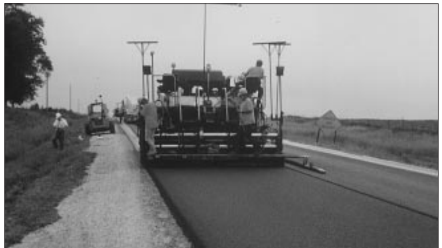
A portion of Iowa 175 in Hardin County, Iowa, was constructed in 1995 using Superpave specs.
