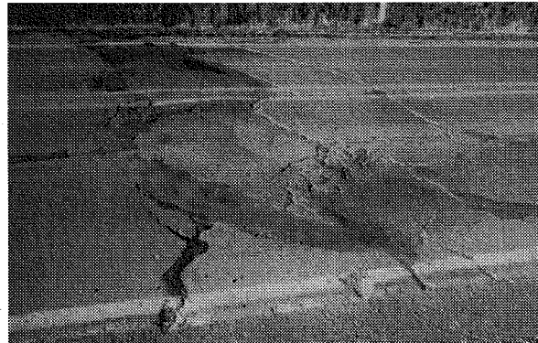
Rubblization is an alternative treatment for severely deteriorated PCC road, like this one in Mills County shown before rehabilitation in 1989.
