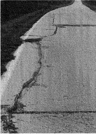
Rubblization is an alternative treatment for severely deteriorated PCC road, like this one in Mills County shown before rehabilitation in 1989.
