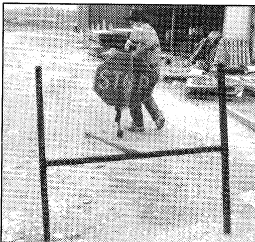
Rick Renataries, a traffic signal technician for West Des Moines, shows how his department's portable stop sign is assembled (left photo). The sign can be put together (right photo) in minutes.
