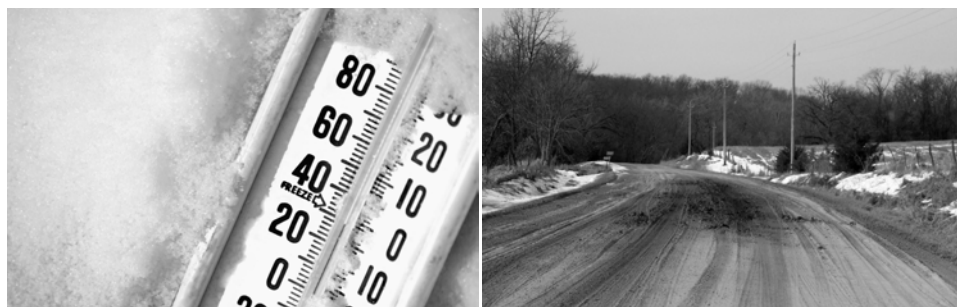
As freezing temperatures begin to climb, roads thaw and frost boils begin to appear
