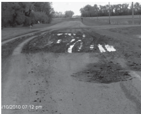
(L) A badly deteriorated low-volume paved roadway in SD that might be a candidate for de-paving (R) Deuel Co. (SD) road turned back to gravel in mid-1980s; photo taken August 2010 (photos courtesy of SD LTAP)
