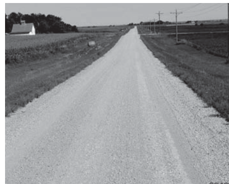
(L) A badly deteriorated low-volume paved roadway in SD that might be a candidate for de-paving (R) Deuel Co. (SD) road turned back to gravel in mid-1980s; photo taken August 2010 (photos courtesy of SD LTAP)
