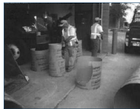
Figure 4. In-house construction of culvert
