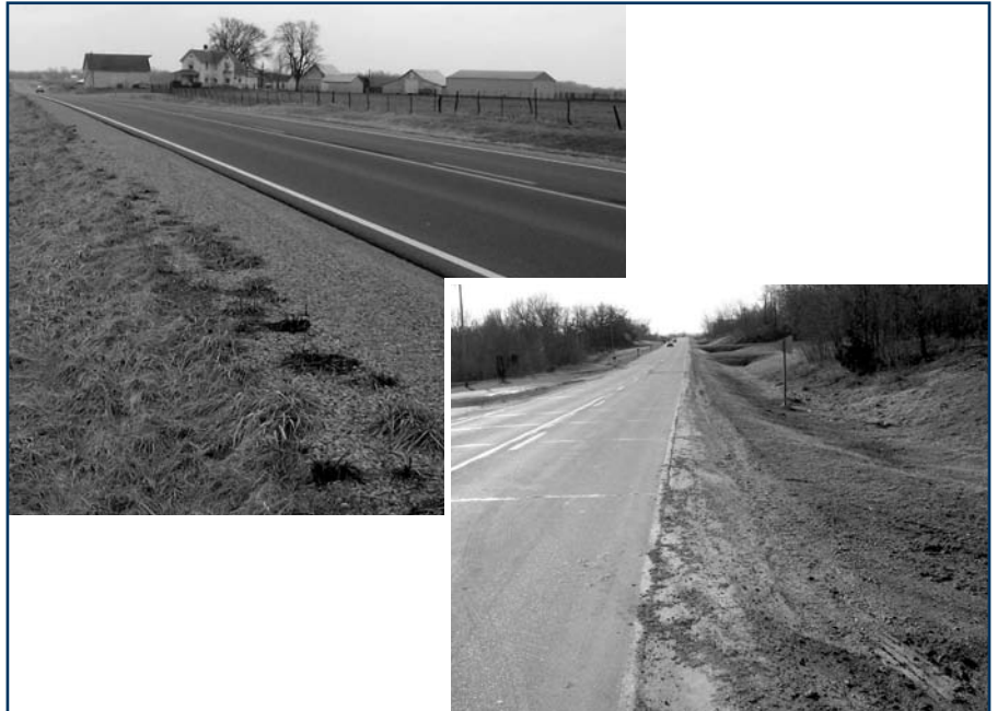
Mowed rights-of-way: flat and level terrain (left) and a typical county road ditch (right) (Unless noted, all photos courtesy of Bob Sperry, Iowa LTAP)
