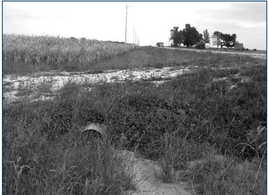
A flattened entrance slope with a culvert
