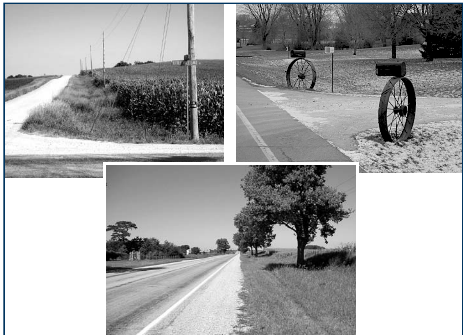
Examples of hazards in clear zone that can affect crash severity (Photos courtesy of Jack Latterell)
