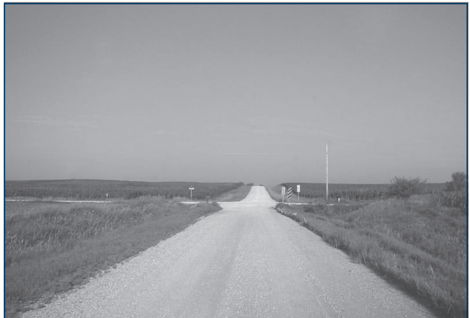
Ultra-low-volume unpaved rural intersections like this one may not need stop signs
