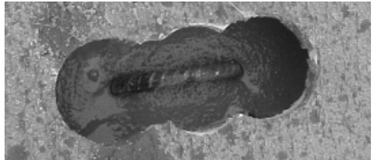
Top: Unlike concrete that must be formed on-site, FRP deck slabs are preformed and transported directly from the factory. Middle: The FRP deck is grouted to shear connectors attached to the bridge girders.
