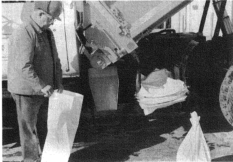
Photo 1 – The City of Clive has adapted its dump trucks to fill sand bags.
