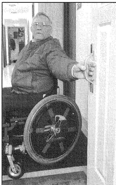
Don Denning uses a passenger assist handle to easily pull a door closed after entering the Warren County annex building in Indianola.
