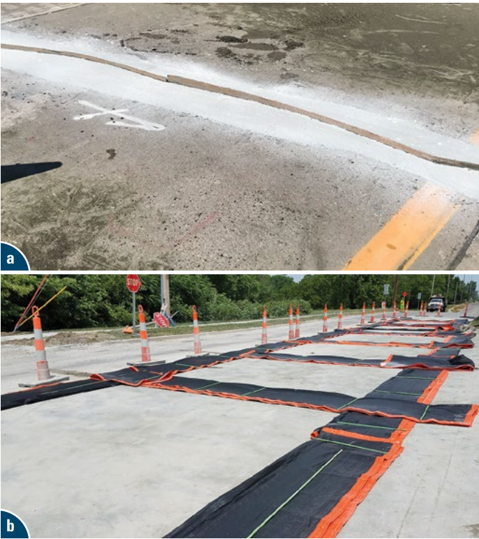
Figure 19. Use of (a) curing agent and (b) insulating blankets for PDRs
