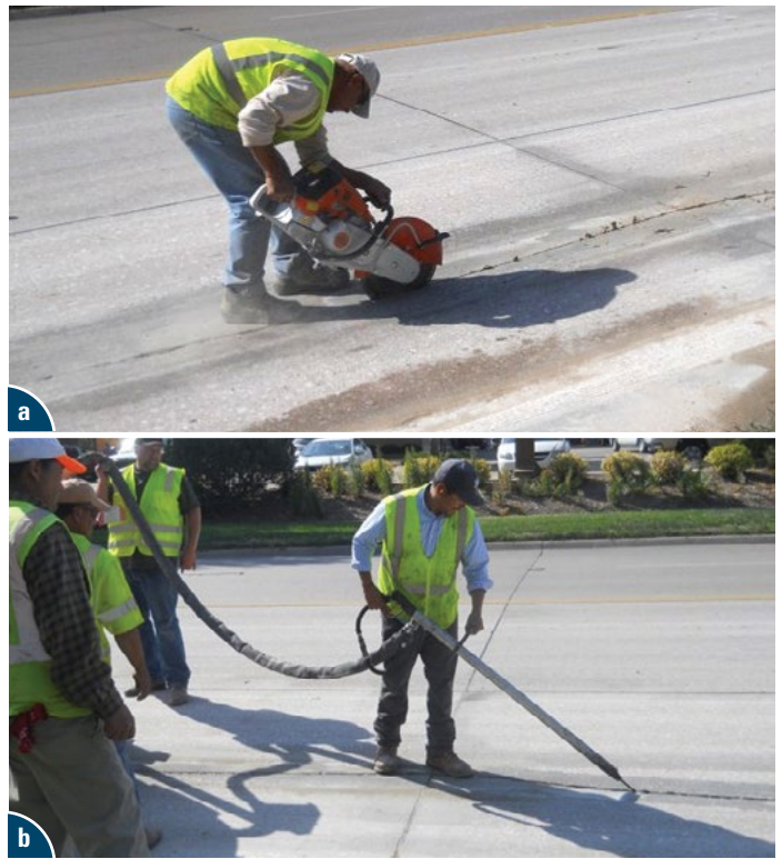
Figure 20. Sawing compression relief material and sealing a PDR
