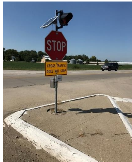
Figure 1. Flashing beacon mounted to a stop sign
