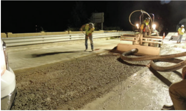
Figure 6. Hydrodemolition resulting in concrete slurry prior to removal from bridge deck
