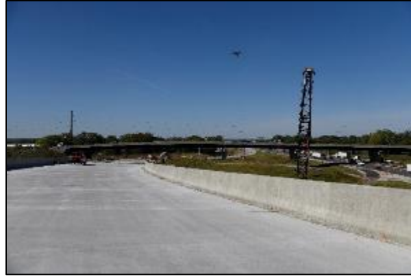
Figure 13. sUAS being navigated near the edge of the bridge to ensure that all target areas are covered precisely
