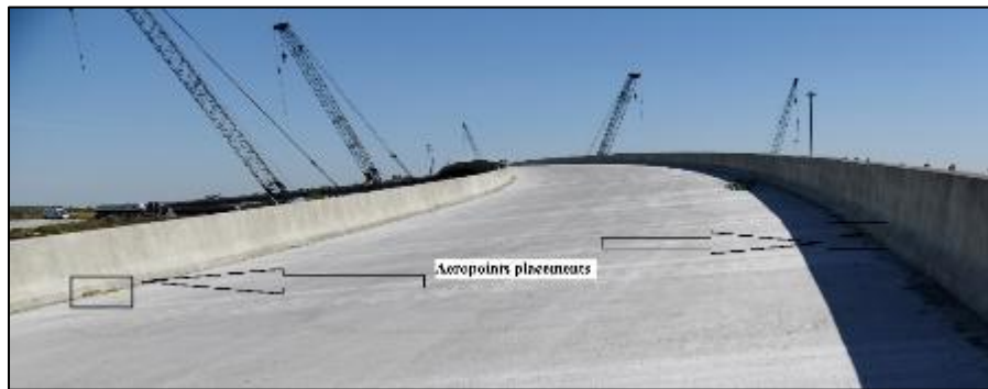
Figure 8. Placement of AeroPoints GCPs on the ground
